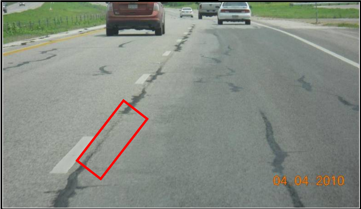
Category 1: US 90 from west of SL 1604 to Bexar county line (long. cracking and poor ride)
