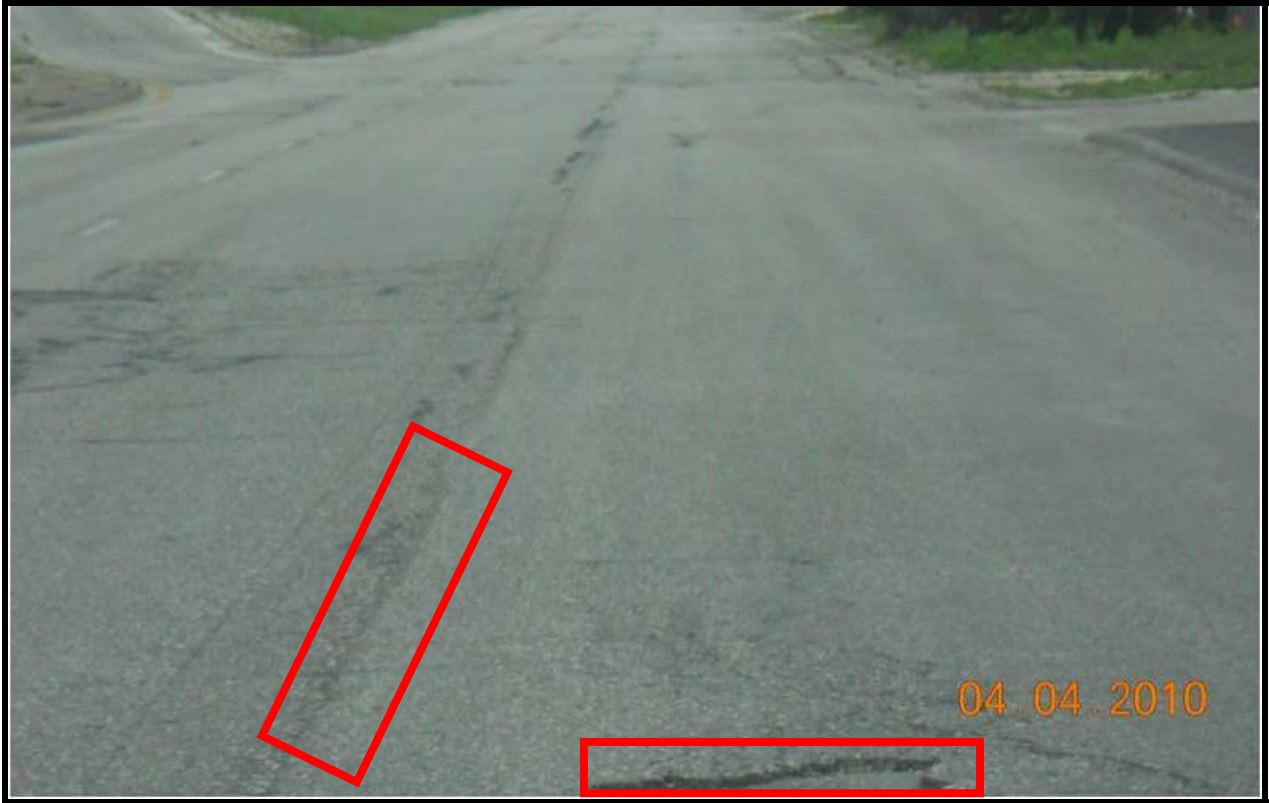
Category 4: IH 410 SB+NB FR from FM 78 to Rittiman (potholes and long. and trans. cracking)
