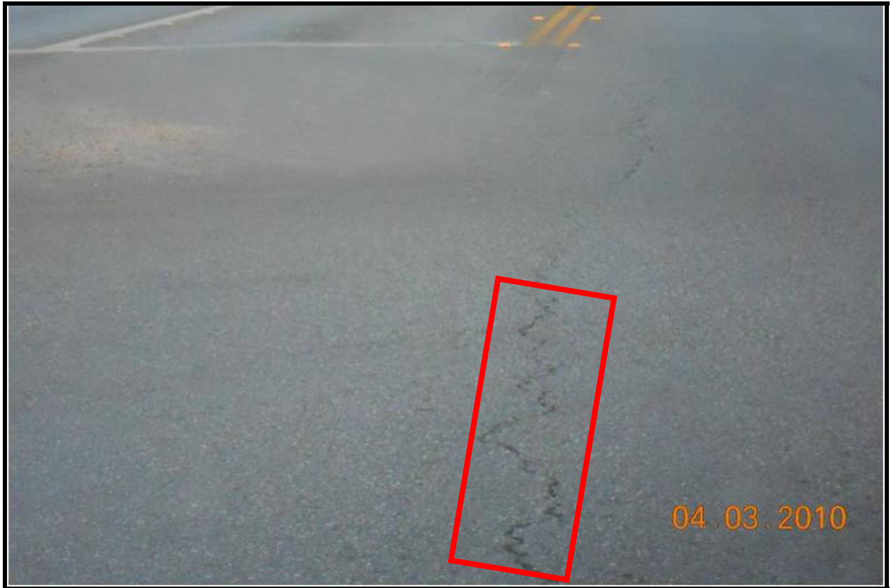
Category 7: FM 758 from Guadalupe county line to FM 78 (long. cracking and raveling)
