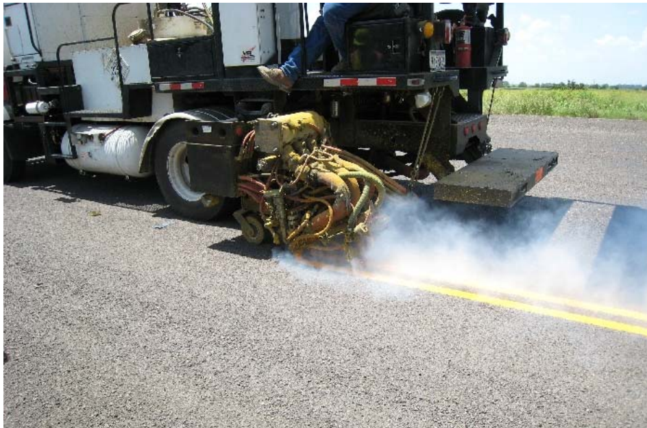
Figure 9. SH 21 Lead-Free Thermoplastic Installation.
