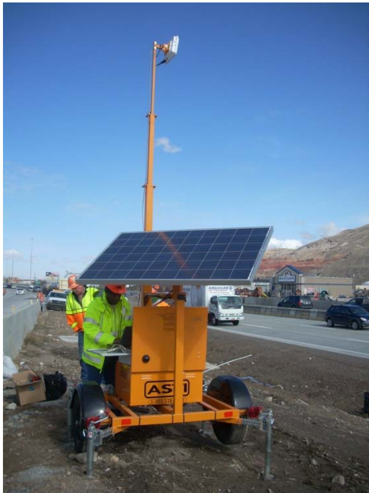
Figure 3-3 Final location for sensor 5 (taken by Mitsuru Saito).
