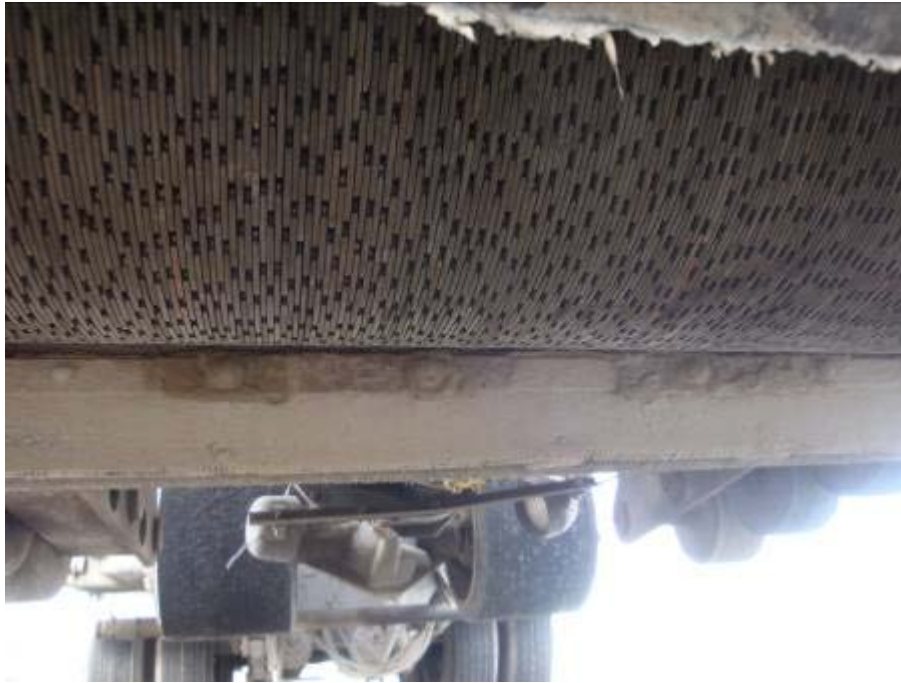
Figure 7. Grinding head for the first pass flush grind operation.
