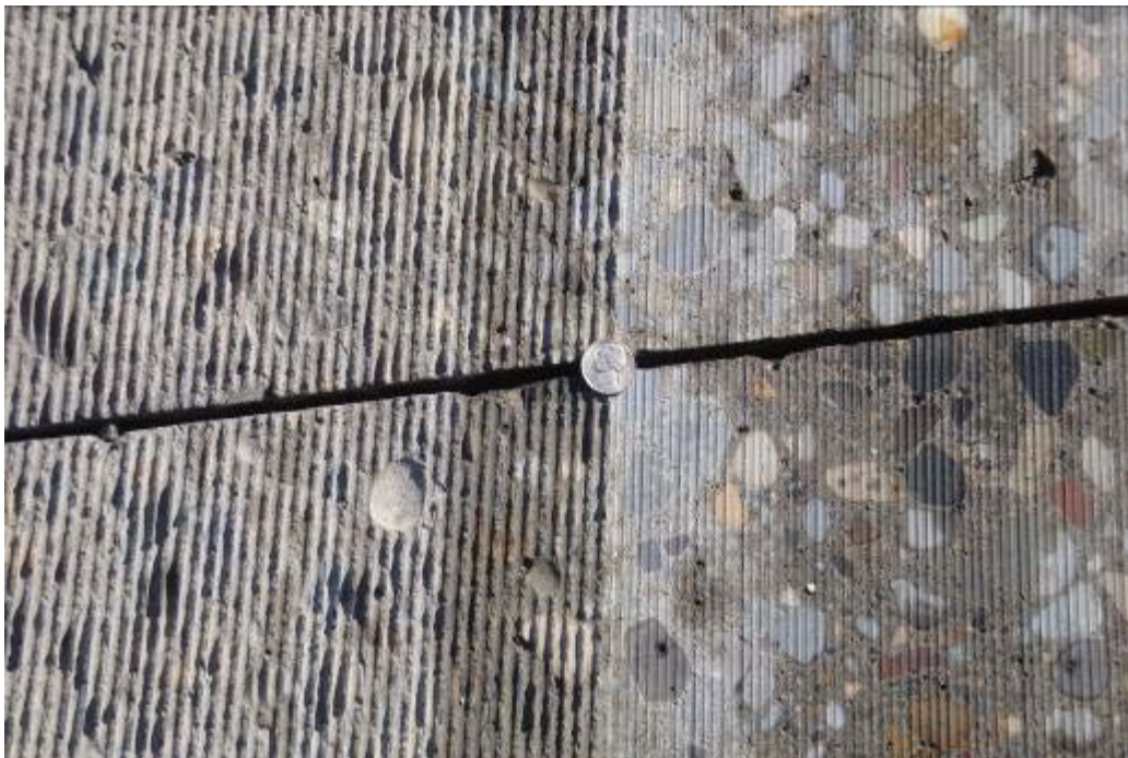
Figure 9. Conventional diamond ground surface on the left, fine flush grind surface of the NGCS first pass operation on the right.
