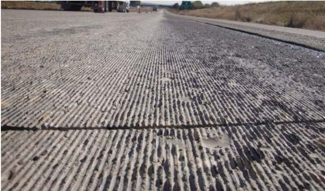
Figure 15. Roadway surface after conventional grinding.
