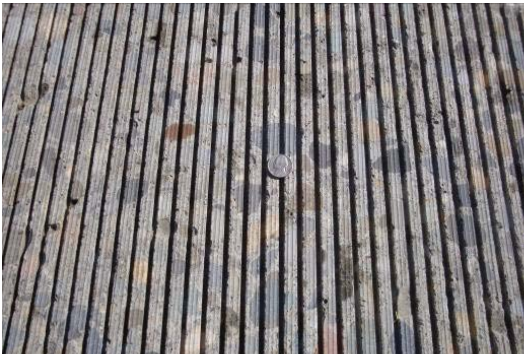
Figure 12. Finished surface of the NGCS with wide, flat land areas and deep grooves.
