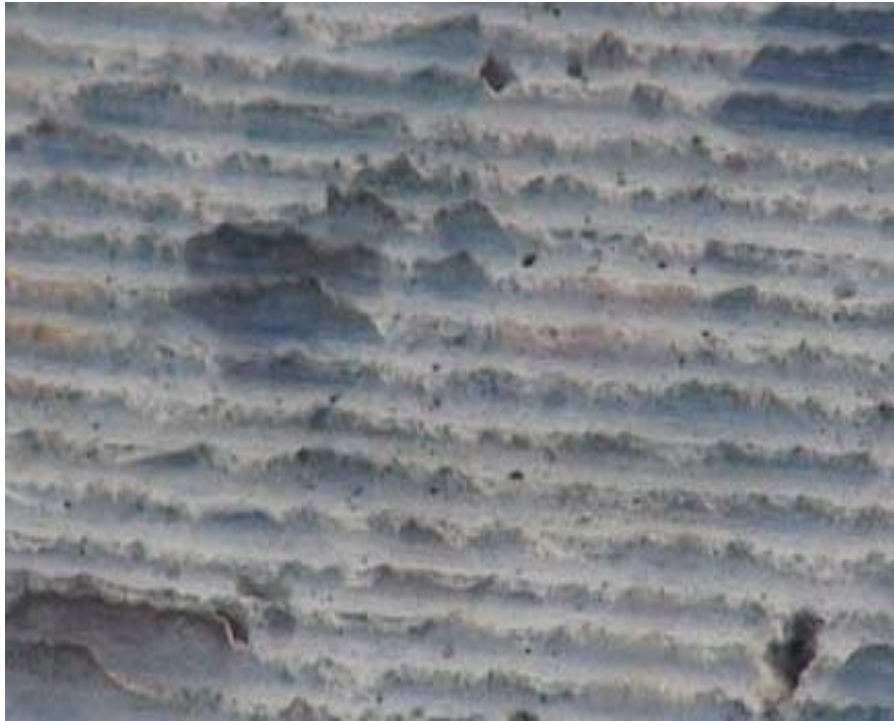
Figure 2. Positive fin texture produced by conventional diamond grinding. (1)
