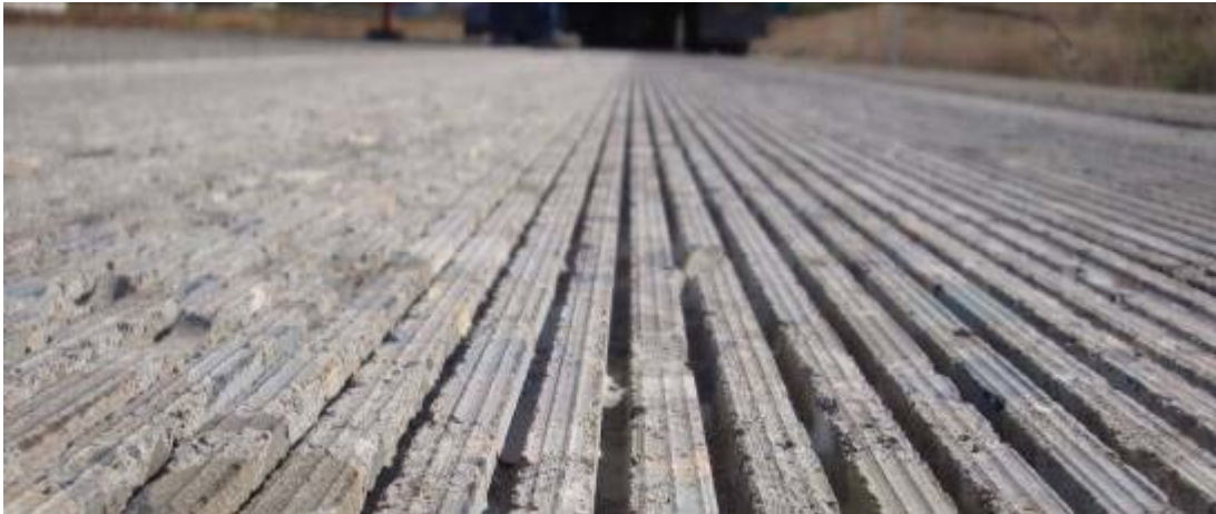
Figure 19. Pavement surface after tall blade grinding.
