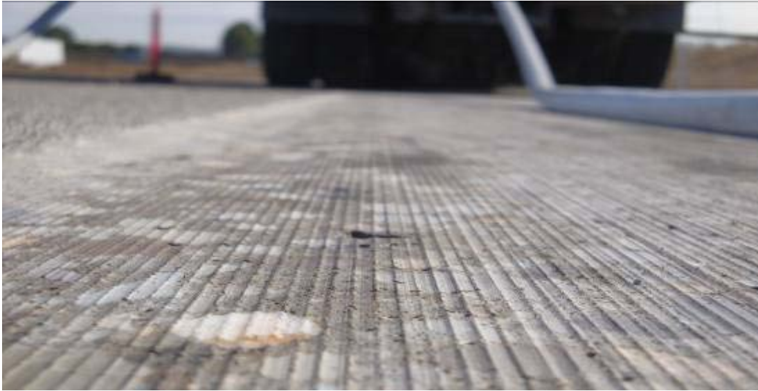
Figure 17. Pavement surface after fine grinding.
