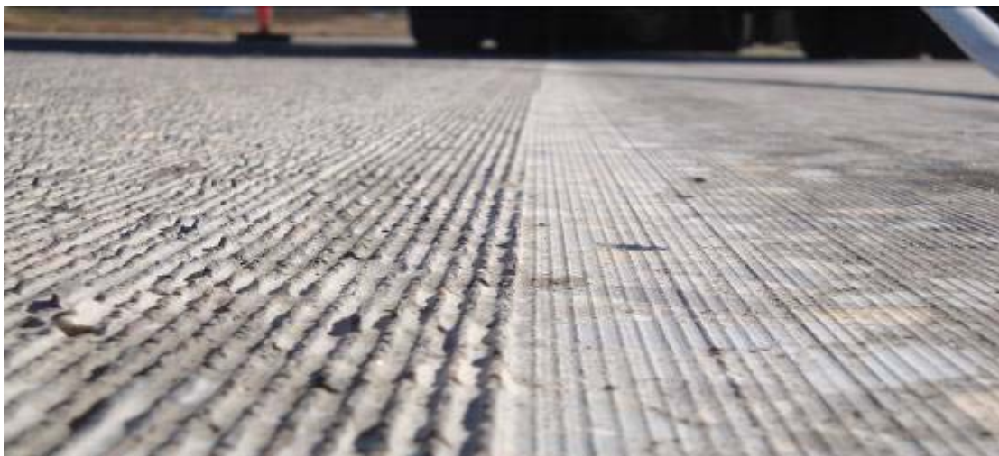
Figure 20. Conventional diamond grind on left with fine grind of NGCS on right before grooves were cut.
