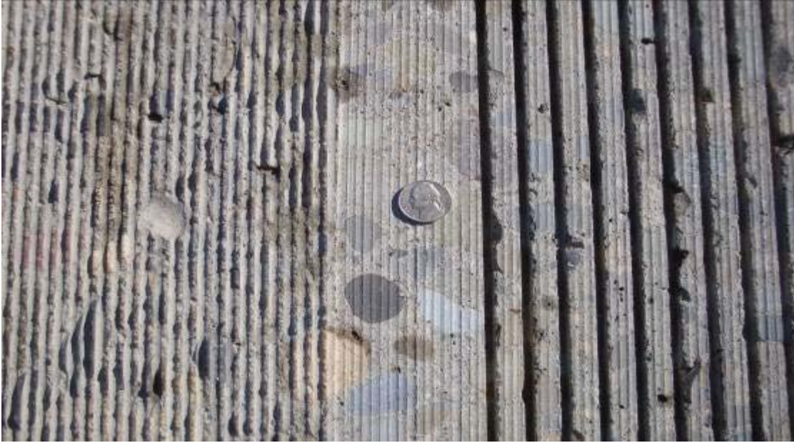
Figure 21. Conventional grind on left, fine grind in middle, and tall grind (complete NGCS) on right.
