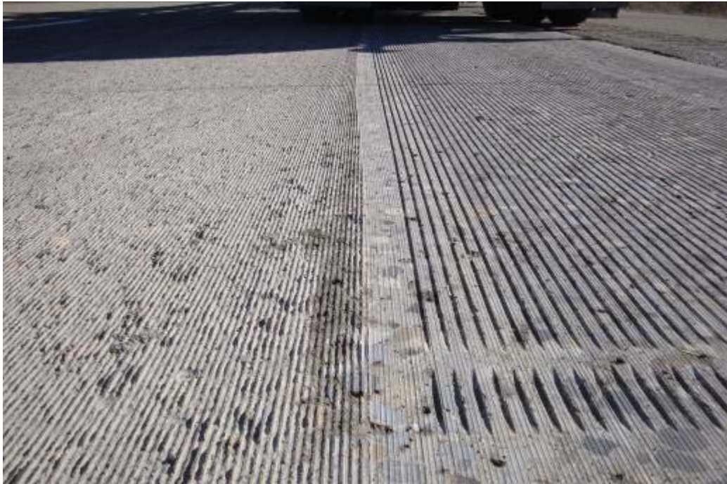
Figure 11. Conventional diamond ground surface on the left, first pass of NGCS in the middle and final pass of the NGCS on the right.
