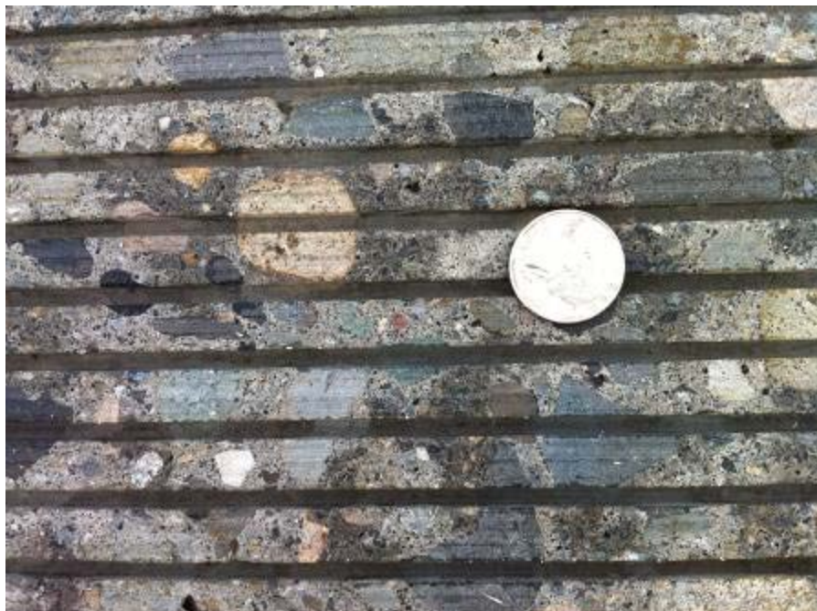
Figure 3. NGCS on I-82 with flat land surfaces and negative grooves
