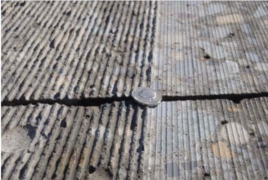
Figure 10. Close-up of the CDG surface on the left and the, first pass of the NGCS on the right.
