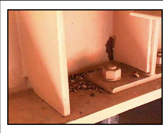
Figure 23. Moderate Damage: Crack in web of steel girder. Note that this may be a red flag condition if it is in the primary member. (CPHMR)
