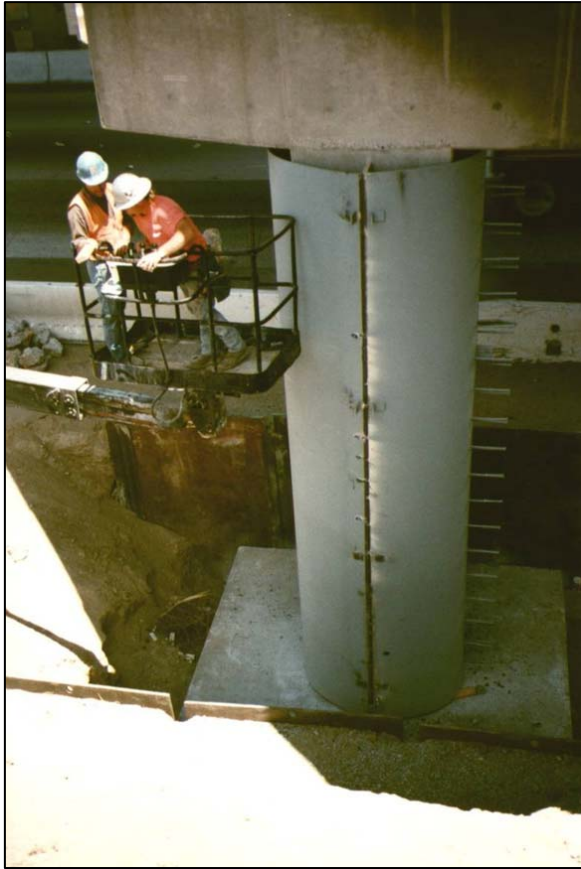
Figure 64. Seismic retrofit of a bridge column using a steel jacket (Aboutaha, 1994)
