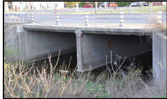
Figure 81. Concrete Box Culvert
