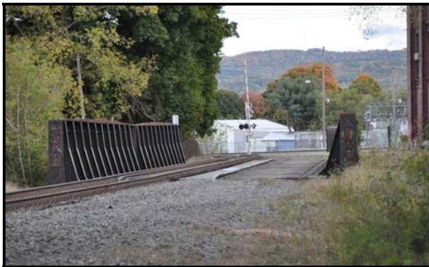
Figure 82. Thru-Girder
