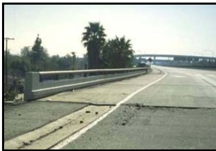
Figure 8a. PBDA Column #1 Approach
