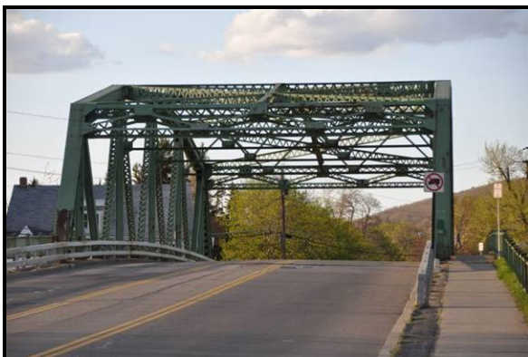
Figure 76. Steel Through Truss
