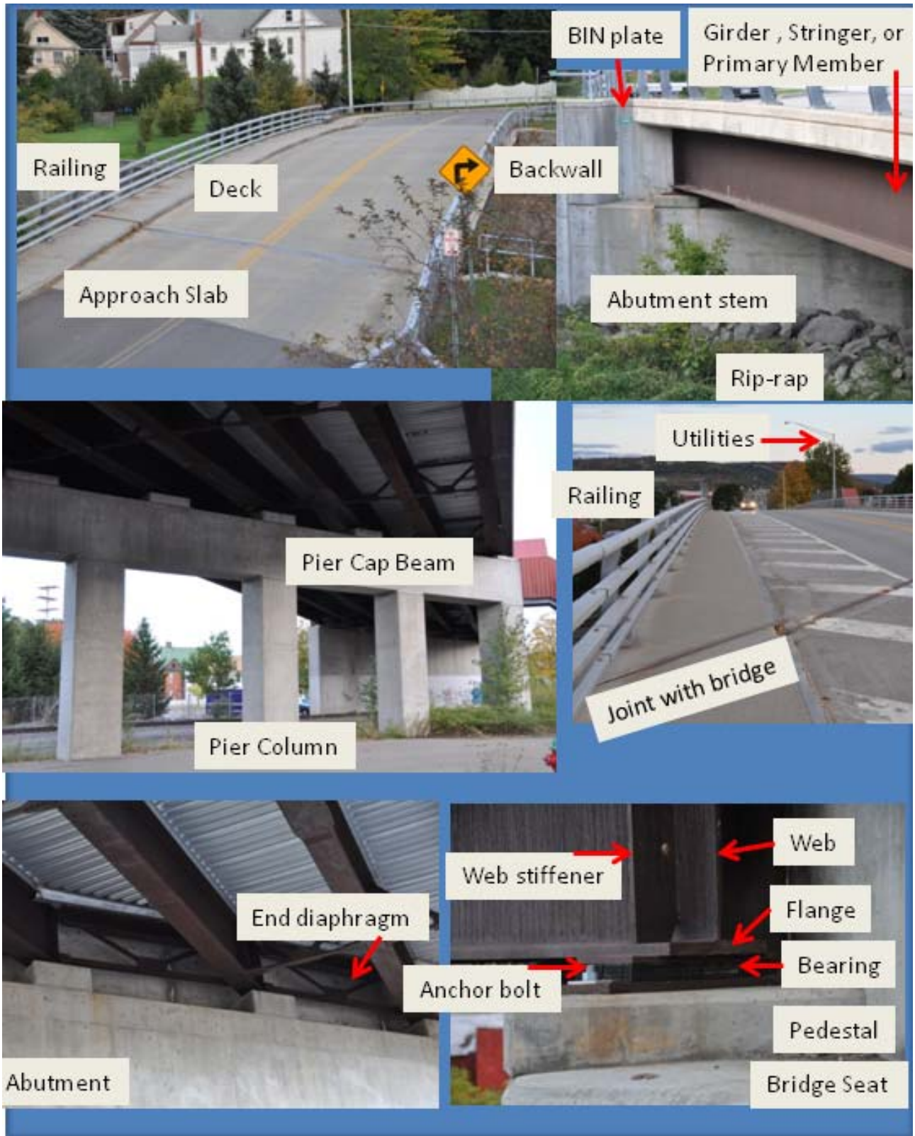
Figure 71. Bridge Terminology Reference Sheet
