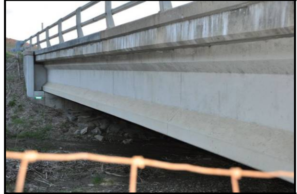
Figure 73. Pre-Stressed Concrete Girder
