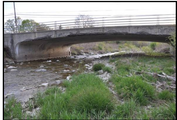
Figure 75. Reinforced Concrete Arch
