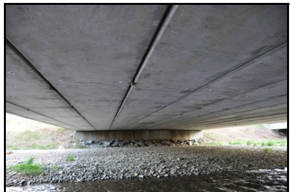
Figure 77. Adjacent Prestressed Concrete Box Beams (O'Connor)
