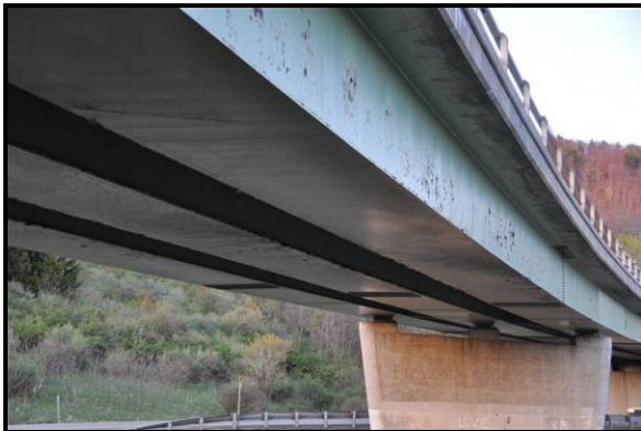
Figure 74. Steel Box Girder
