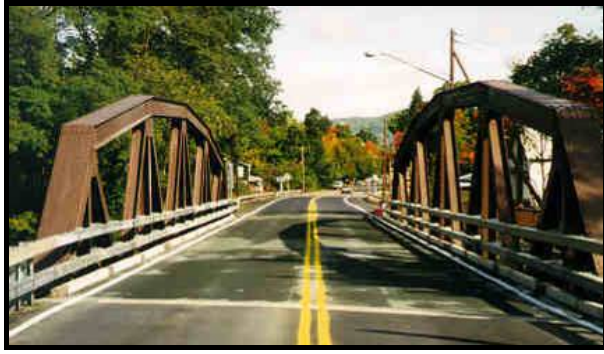
Figure 78. Steel Pony Truss
