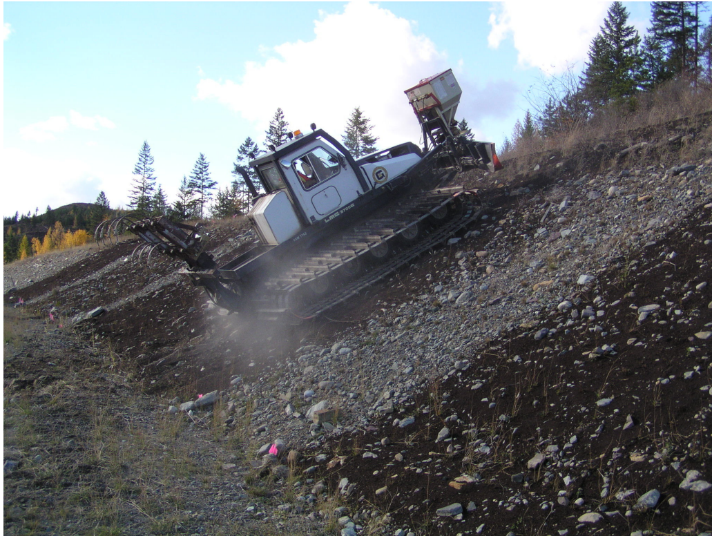
Figure 20. Modified LMC 3700C initiating tillage on plot 8, MP 69 site.
