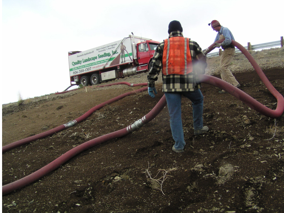
Figure 23. Express Blower (Rexius) blower truck model EB-30 applying Earth Systems compost to Plot 17.
