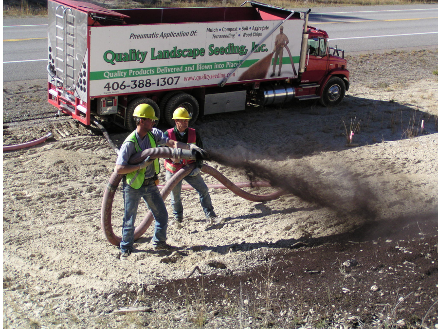
Figure 19. Express Blower Model EB-30 applying compost at the MP 77 site.
