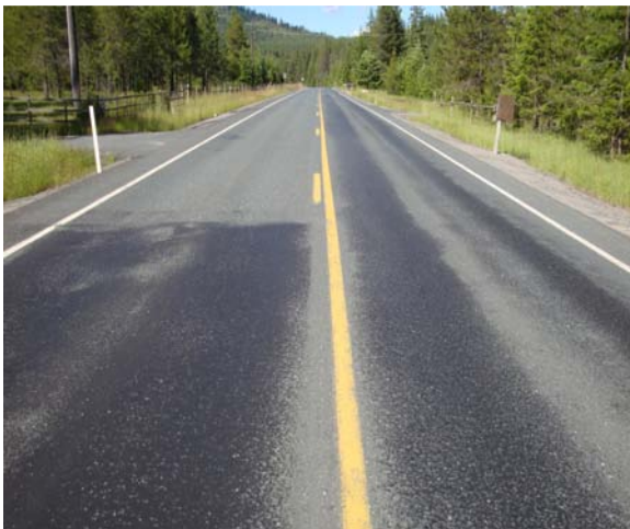
Figure 9. Upper left – Rating 1 (No Flushing), Bottom left – Rating 4 (Entire lane flushing) and Right – Rating 3 (Consistent wheel path flushing).
