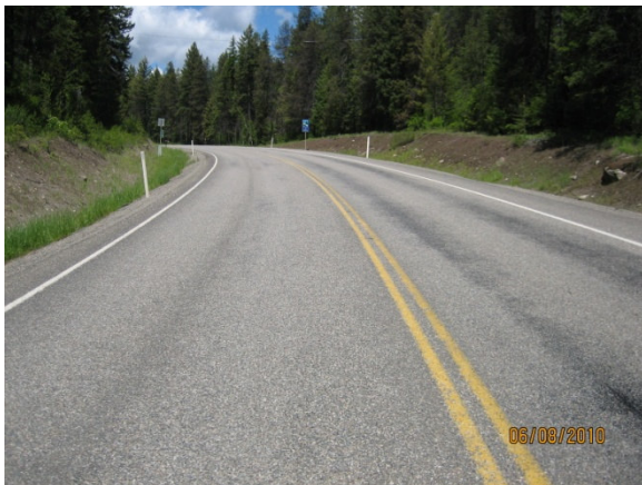
Figure 7. Test Section 4 (on left) with 0.20 gal/sy shows minimal flushing while Test Section 2 (on right) with 0.28 gal/sy shows flushing in wheel paths two years after construction.
