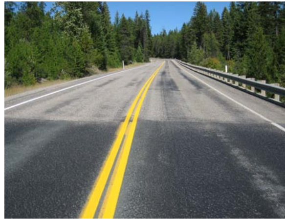
Figure 6. East end of Test Section 4 (on the left) with 0.20 gal/sy and Test Section 2 (on the right) with 0.28 gal/sy for the first application.
