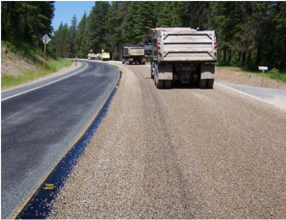
Figure 3. Chip seal placement on Test Section 1 (on right) with 0.27 gal/sy showing slight flushing in the wheel path after the first application.
