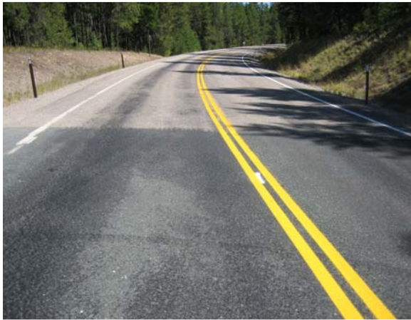
Figure 5. West end of Test Section 1 (on left) with 0.27 gal/sy and Test Section 3 (on right) with 0.20 gal/sy for the first application one year after placement.
