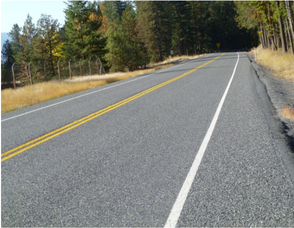
Figure 11. Appearance of the double chip seal two months after construction.
