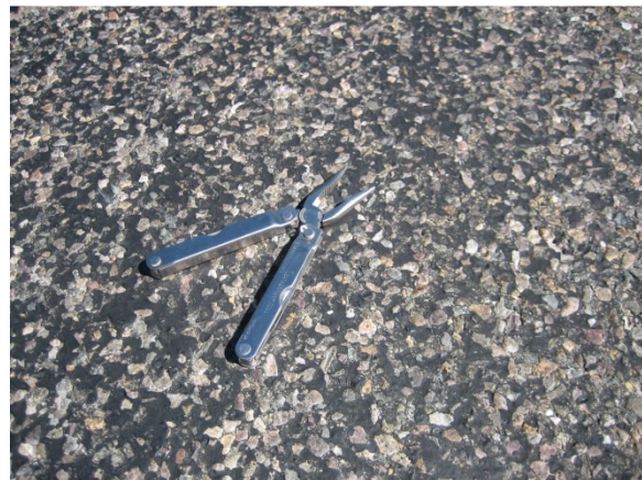
Figure 8. Typical 100% embedment area in Test Sections 1 and 2 one year after construction.
