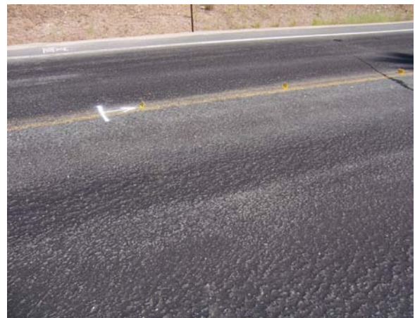
Figure 2. Condition of flushing pavement before placement of the double chip seal.
