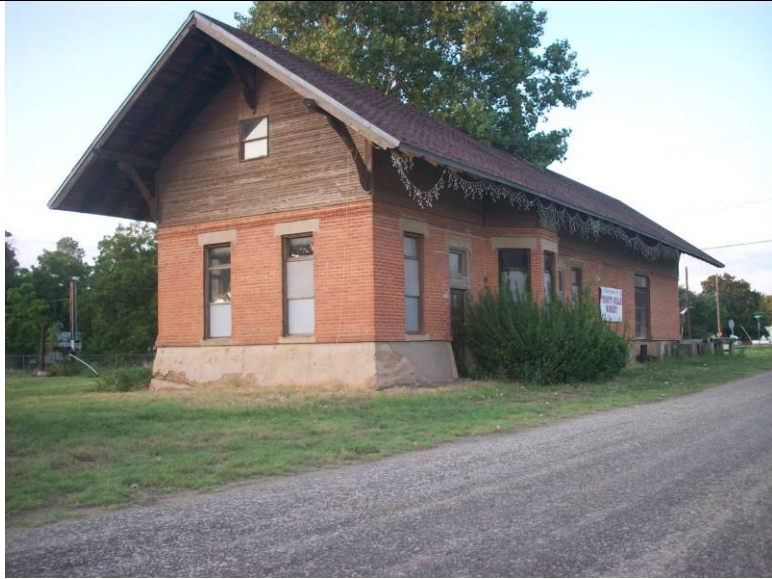
A. Rosser Train Station – located Southeast of Dallas along SH 34
