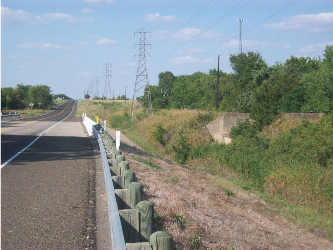
Figure 37. Milford Abandoned Rail Corridor Used for Utility Purposes.
