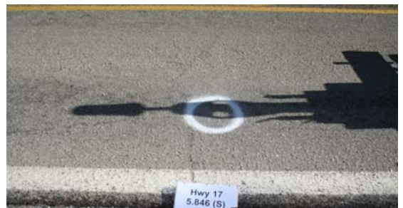
(f) Phase 3-Southbound-Jan 2009
