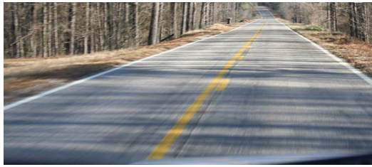
(a) Middle Job Northbound 9 of 16
