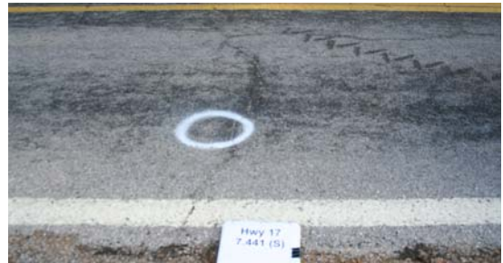
(f) Phase 3-Southbound-Jan 2009
