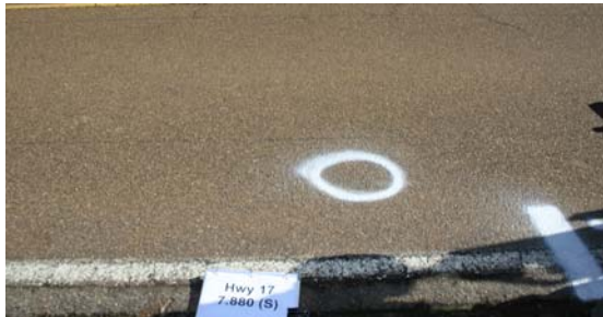
(f) Phase 3-Southbound-Jan 2009
