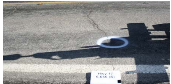
(f) Phase 3-Southbound-Jan 2009
