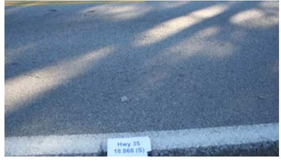
(f) Phase 3-Southbound-Jan 2009
