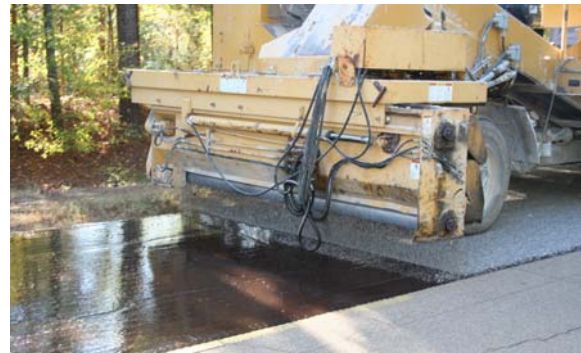
(b) Covering Emulsion w/ Aggregate-Hwy 17
