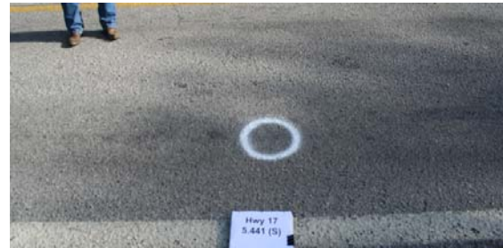
(f) Phase 3-Southbound-Jan 2009
