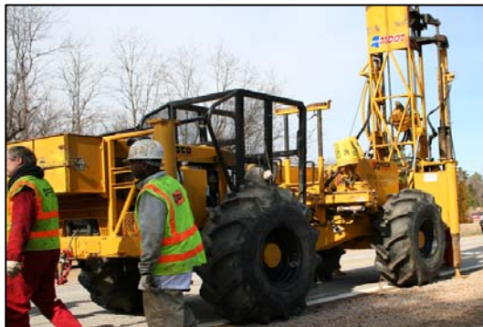
(a) Drilling Equipment Used for Coring
