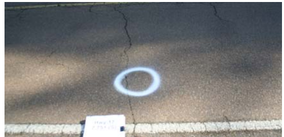
(f) Phase 3-Southbound-Jan 2009
