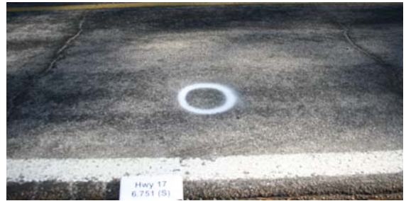
(f) Phase 3-Southbound-Jan 2009
