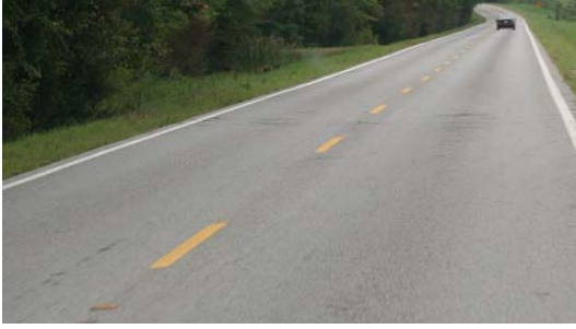
(a) Middle Job Northbound 9 of 16
