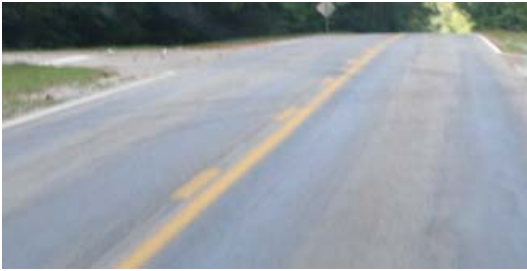
(a) Middle Job Northbound 9 of 16
