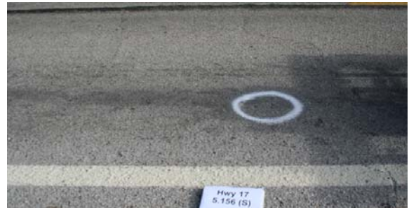
(f) Phase 3-Southbound-Jan 2009
