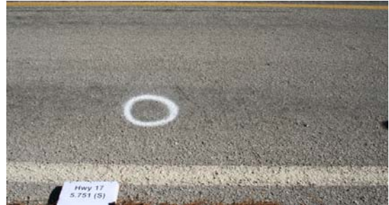
(f) Phase 3-Southbound-Jan 2009
