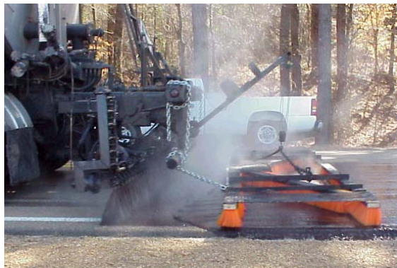
(c) Scrub Seal Emulsion Application-Hwy 35
