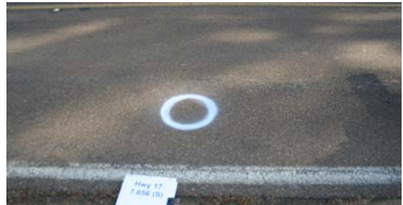
(f) Phase 3-Southbound-Jan 2009
