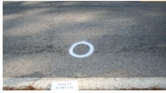
(f) Phase 3-Southbound-Jan 2009
