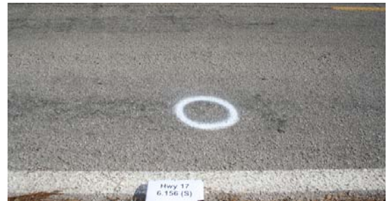
(f) Phase 3-Southbound-Jan 2009
