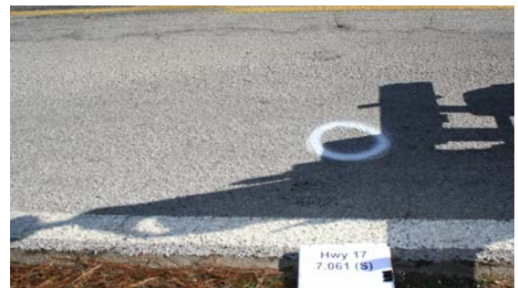
(f) Phase 3-Southbound-Jan 2009
