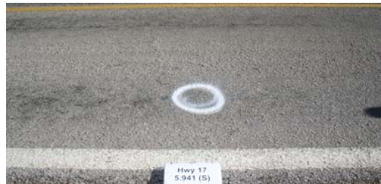
(f) Phase 3-Southbound-Jan 2009
