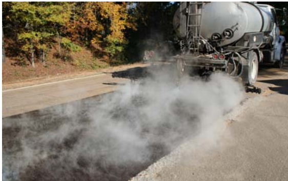
(a) Chip Seal Emulsion Application-Hwy 17
