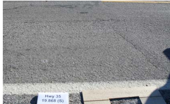
(f) Phase 3-Southbound-Jan 2009
