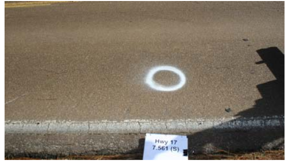
(f) Phase 3-Southbound-Jan 2009
