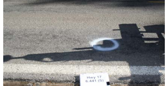
(f) Phase 3-Southbound-Jan 2009
