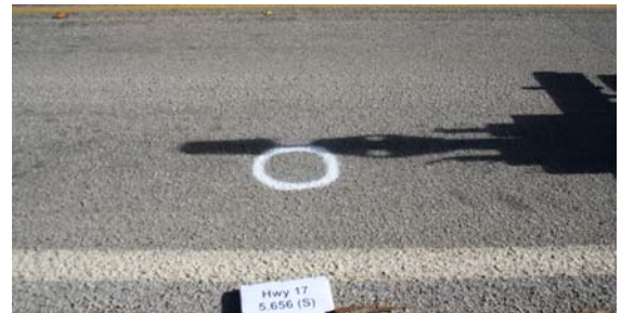
(f) Phase 3-Southbound-Jan 2009
