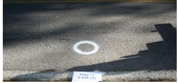
(f) Phase 3-Southbound-Jan 2009
