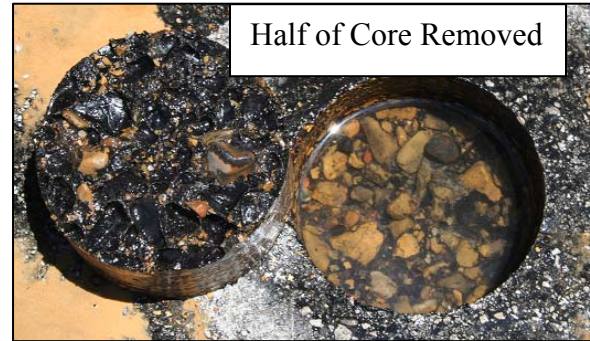
(b) Example of Stripped Core
