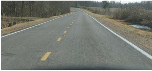
(a) Middle Job Northbound 9 of 16
