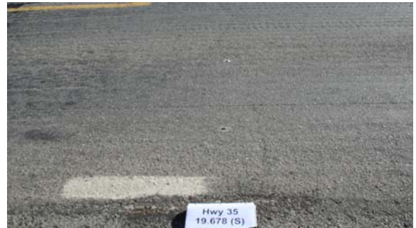
(f) Phase 3-Southbound-Jan 2009
