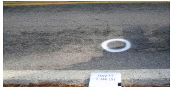
(f) Phase 3-Southbound-Jan 2009
