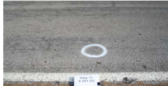
(f) Phase 3-Southbound-Jan 2009
