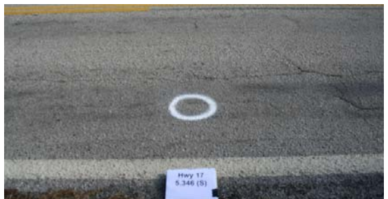
(f) Phase 3-Southbound-Jan 2009
