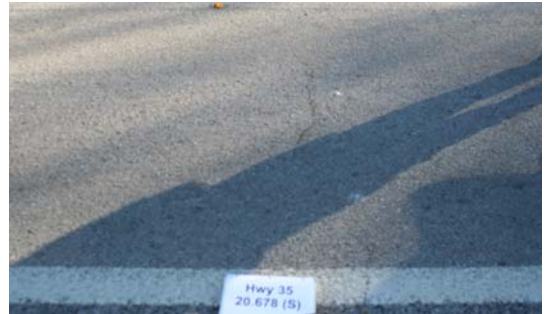
(f) Phase 3-Southbound-Jan 2009
