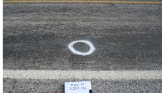
(f) Phase 3-Southbound-Jan 2009
