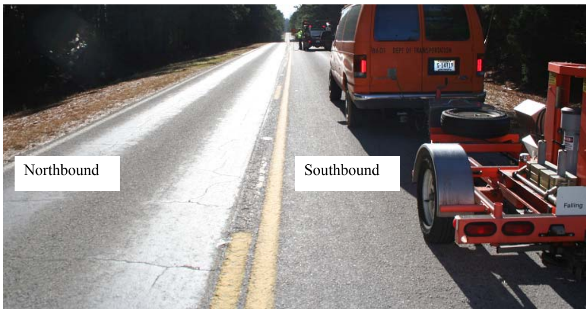
(b) Relative Bleeding/Flushing Photo 2 of 2
