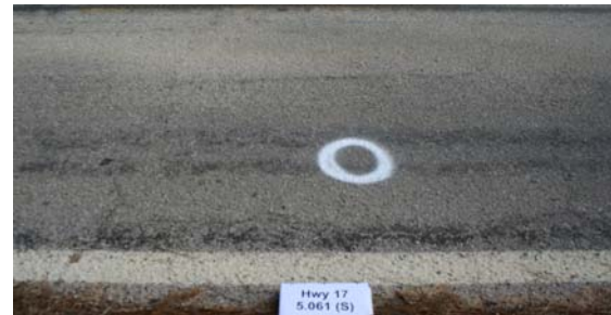
(f) Phase 3-Southbound-Jan 2009
