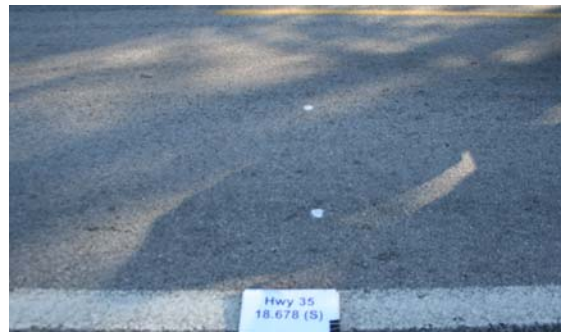
(f) Phase 3-Southbound-Jan 2009
