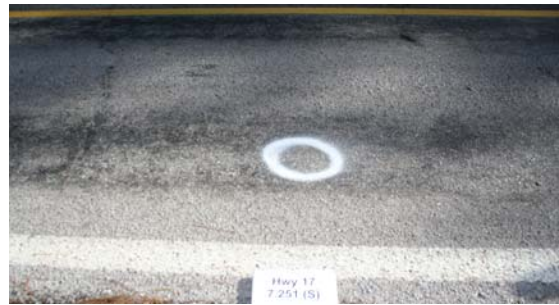
(f) Phase 3-Southbound-Jan 2009
