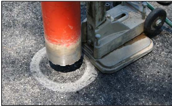
(a) Coring of FWD Test Location
