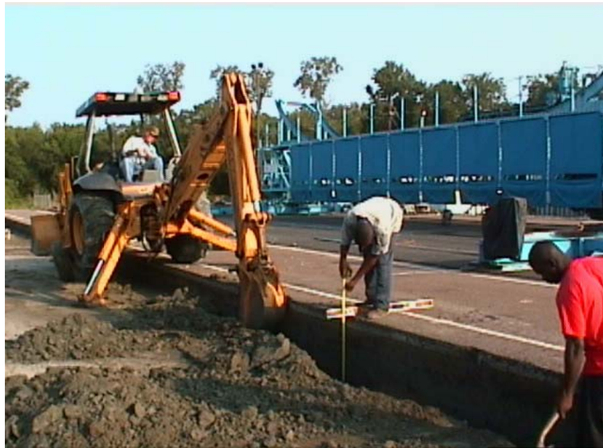
Figure 2 Trench excavation for perforated drain pipe installation
