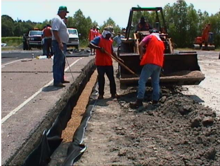
Figure 3 Installation of fabric and backfill
