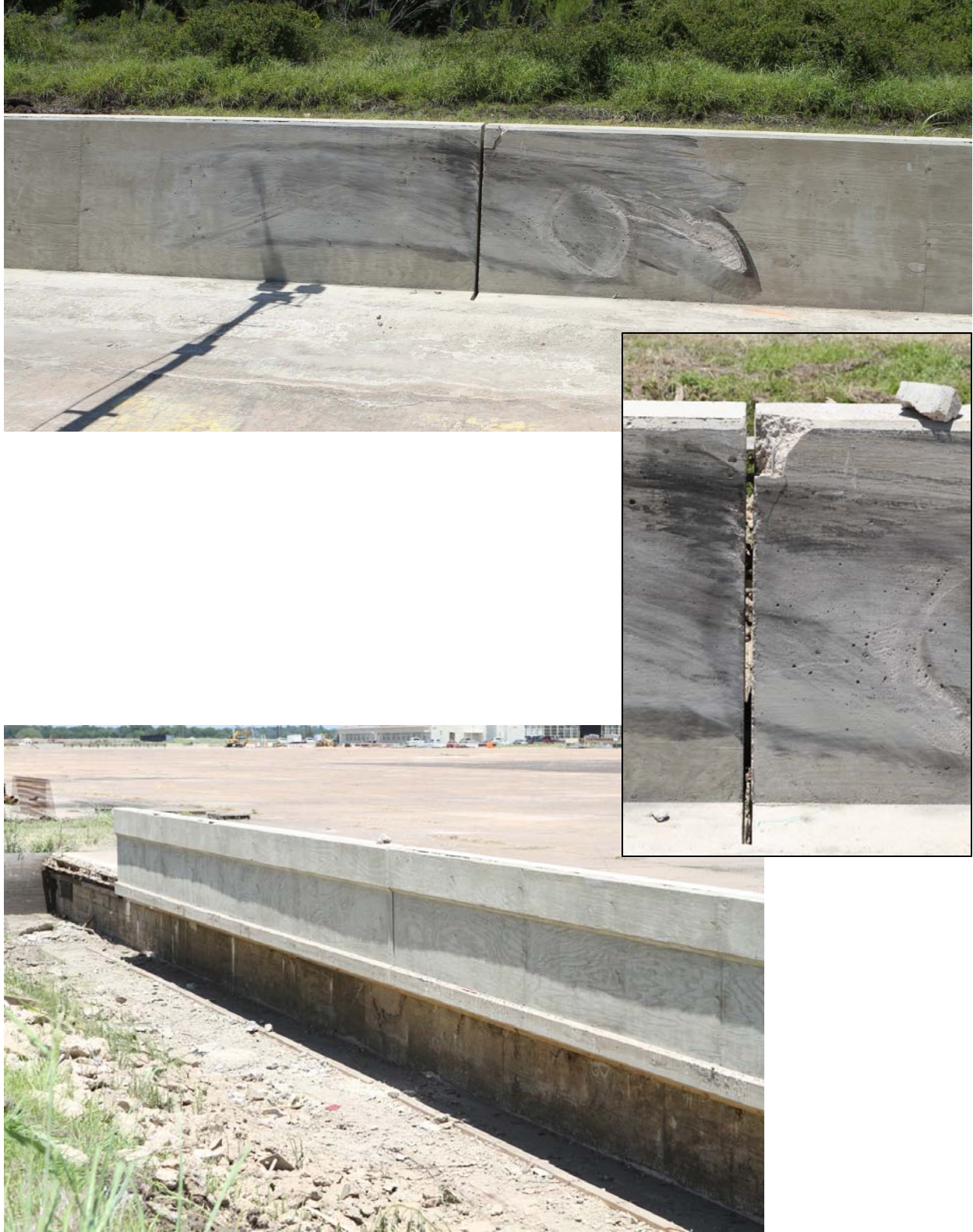
Figure 5.4. Installation after Test No. 420020-3.
