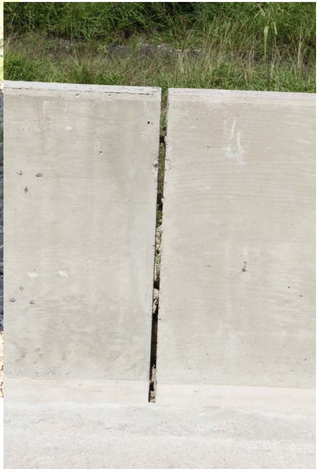
Figure 2.2. TxDOT Pan-Formed Bridge Rail Installation before Test No. 420020-3.
