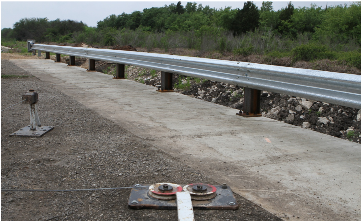
Figure 2.3. T101 Bridge Rail before Test No. 420020-1a.
