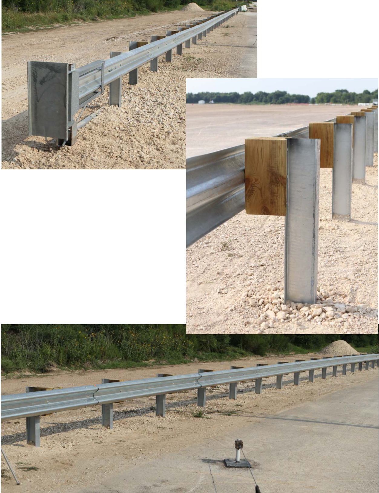
Figure 2.2. Test Article/Installation before Test No. 420020-5.
