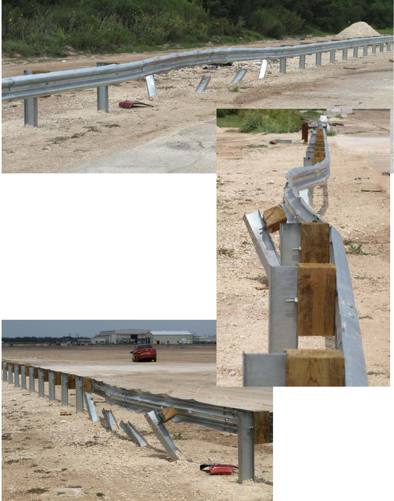
Figure 5.4. Installation after Test No. 420020-5.
