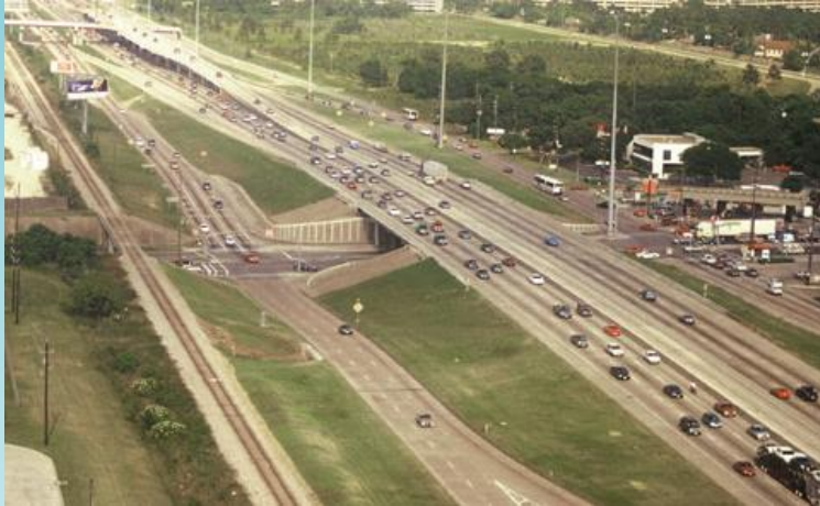
IH10 at SH 6, Before Construction
