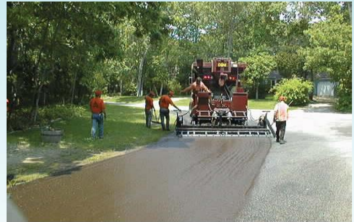
Application of skid-resistant pavement surface in curve.
