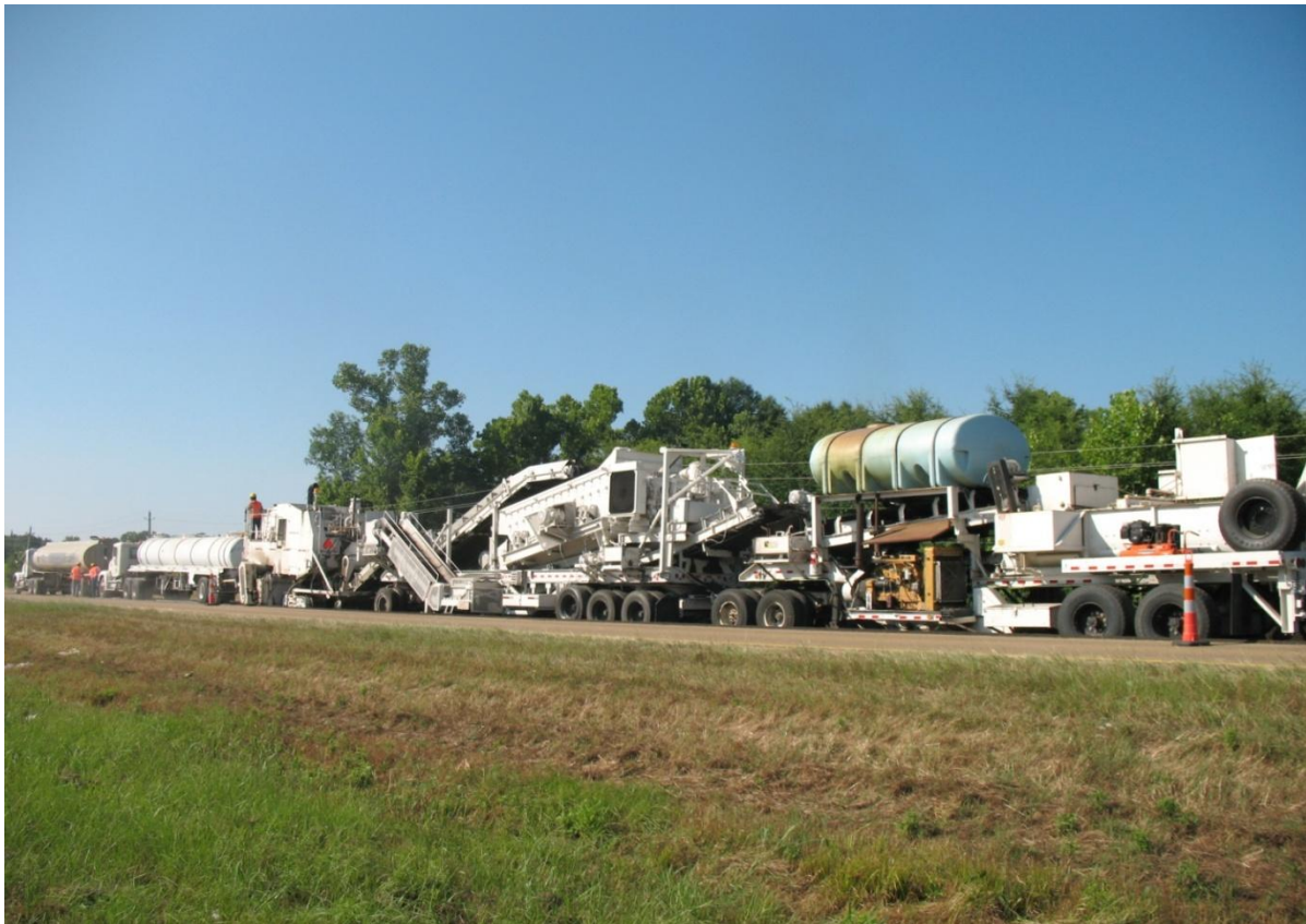
Figure 13: Entire Reclamation Train Assembly
