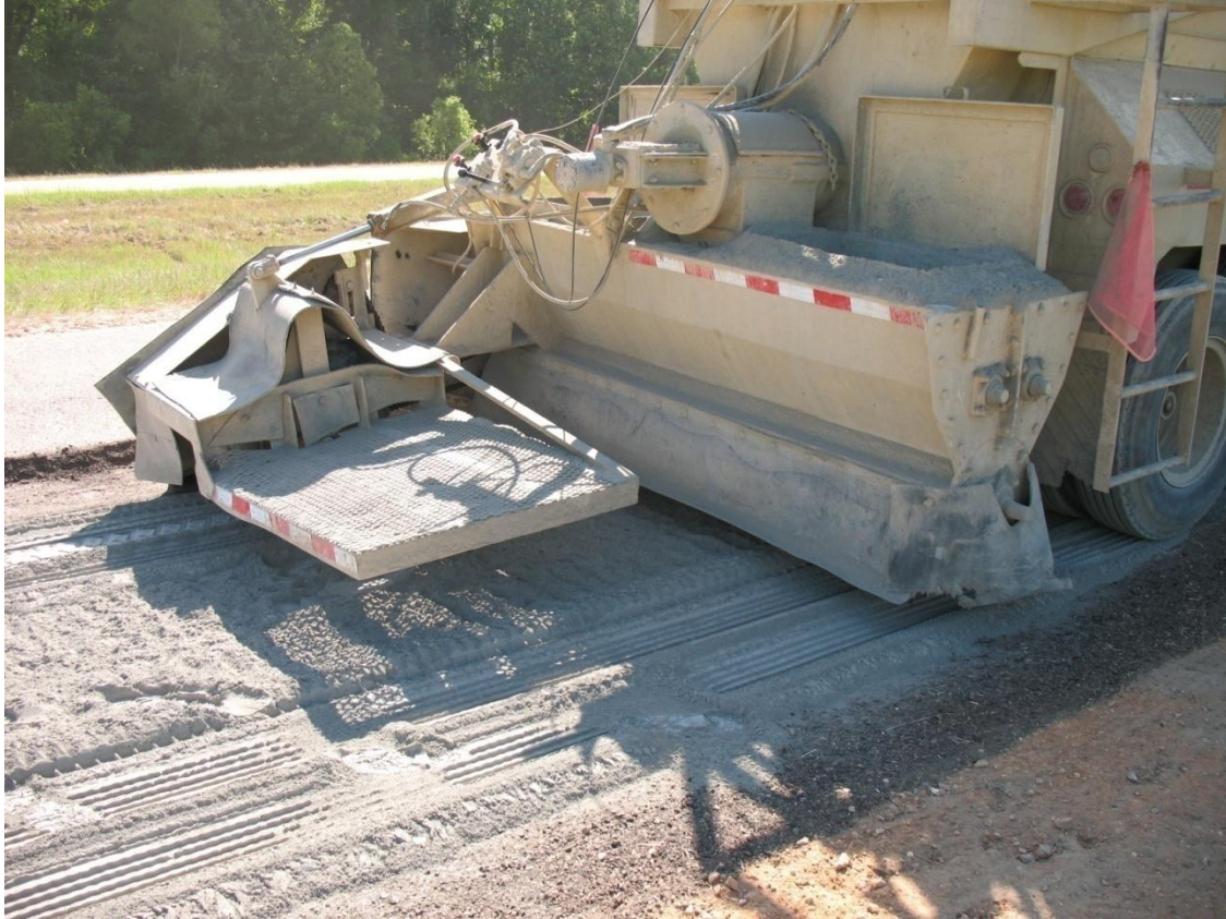
Figure 7: Application of Raw Cement
