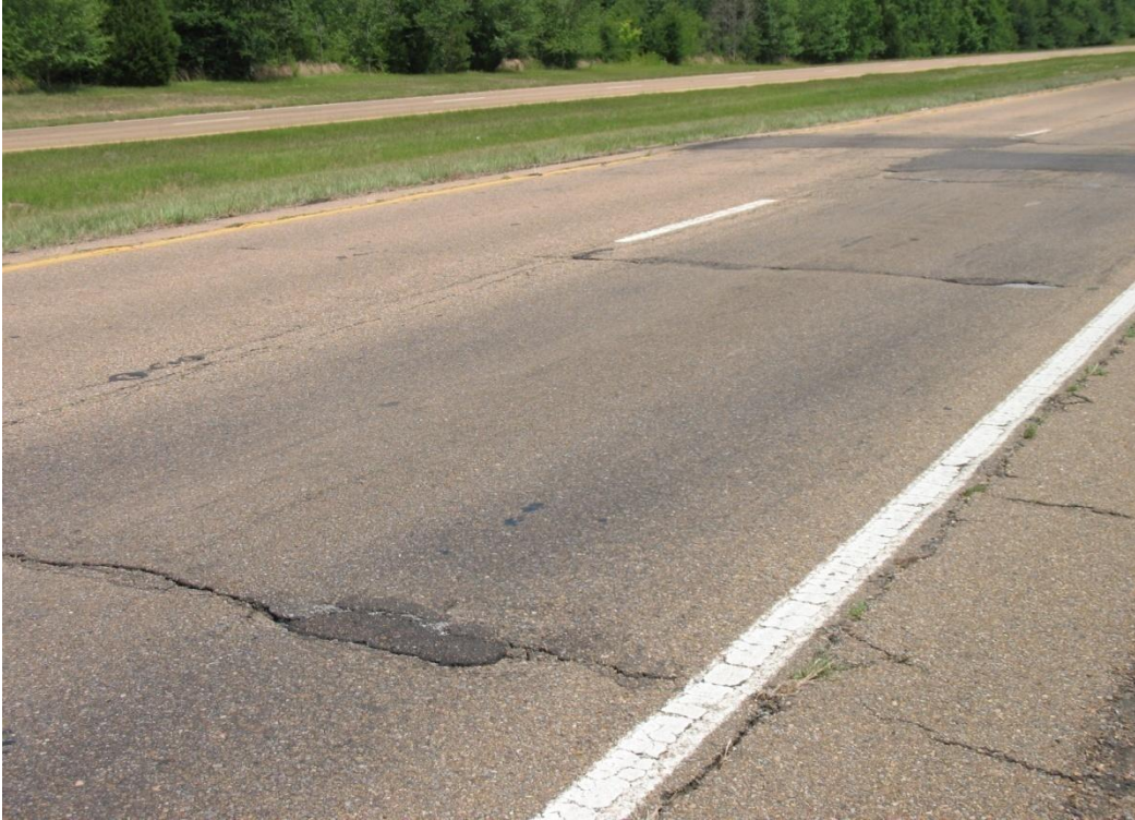
Figure 3: Reflective Cracking
