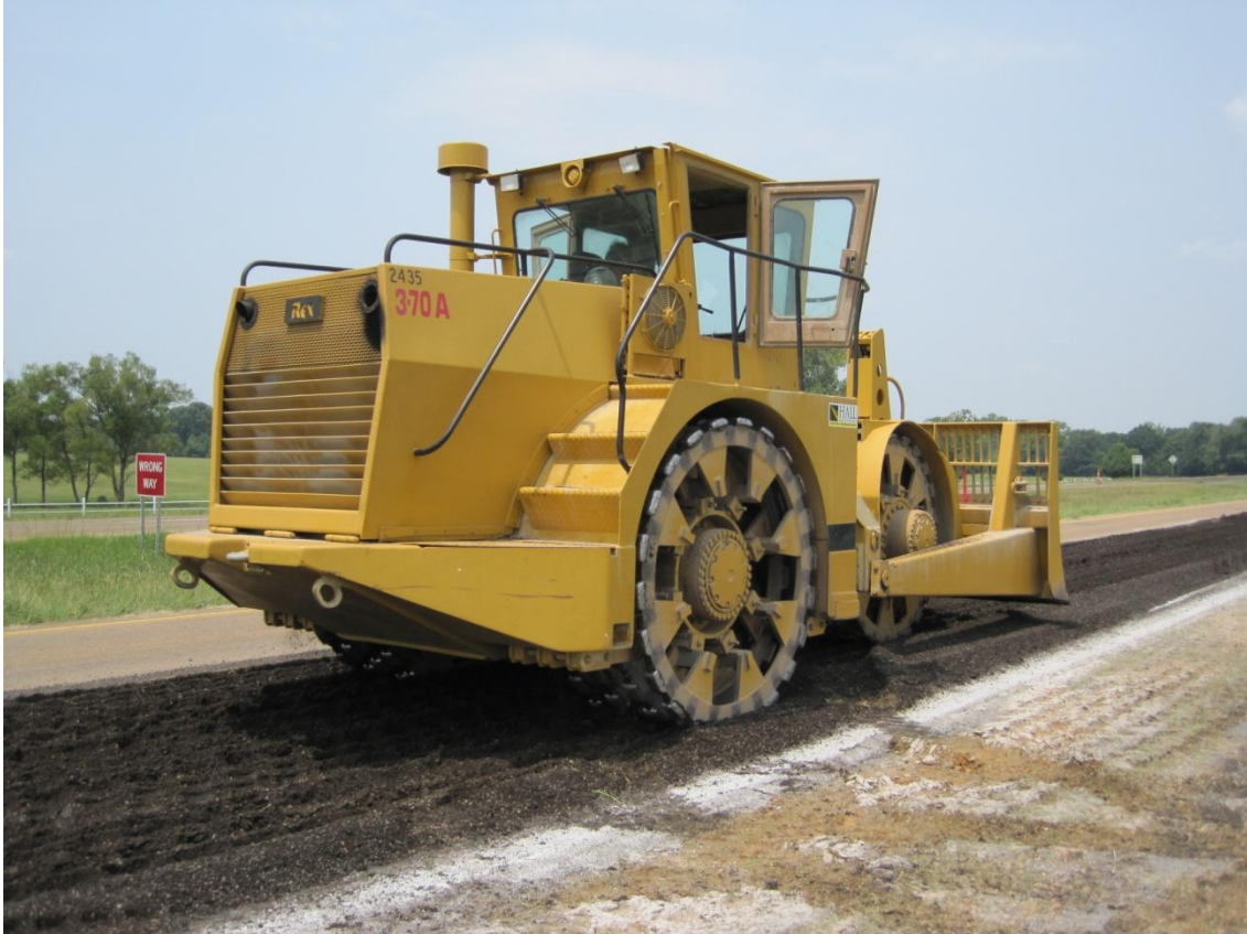
Figure 11: Compaction of Reclaimed Material
