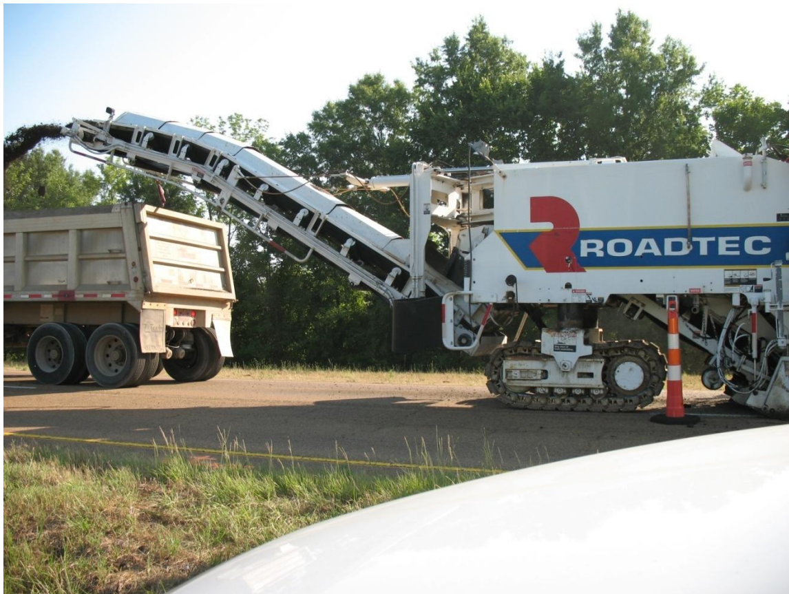
Figure 6: Milling and Surface Removal
