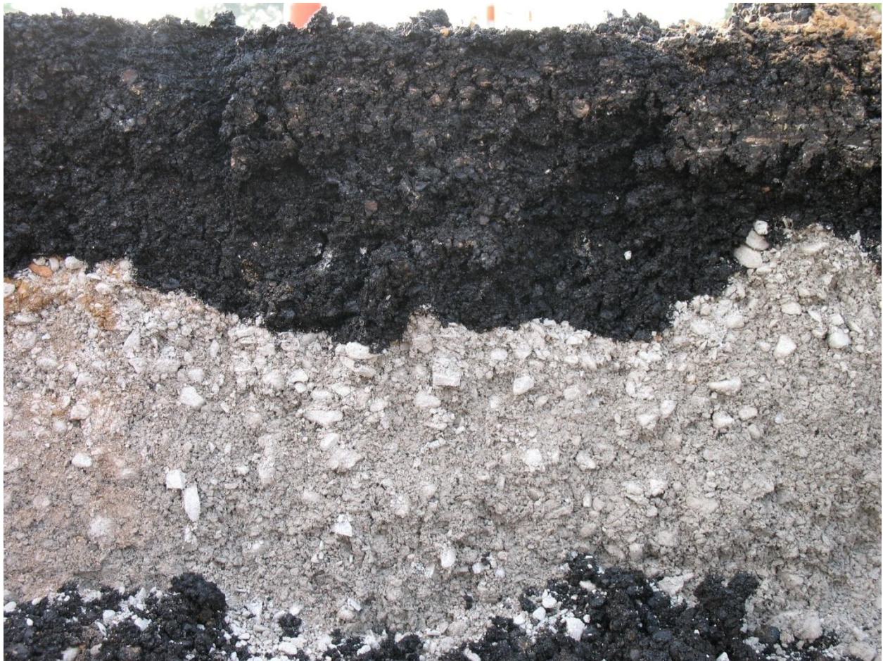
Figure 17: Cross-Section of Reclaimed Layer Repair
