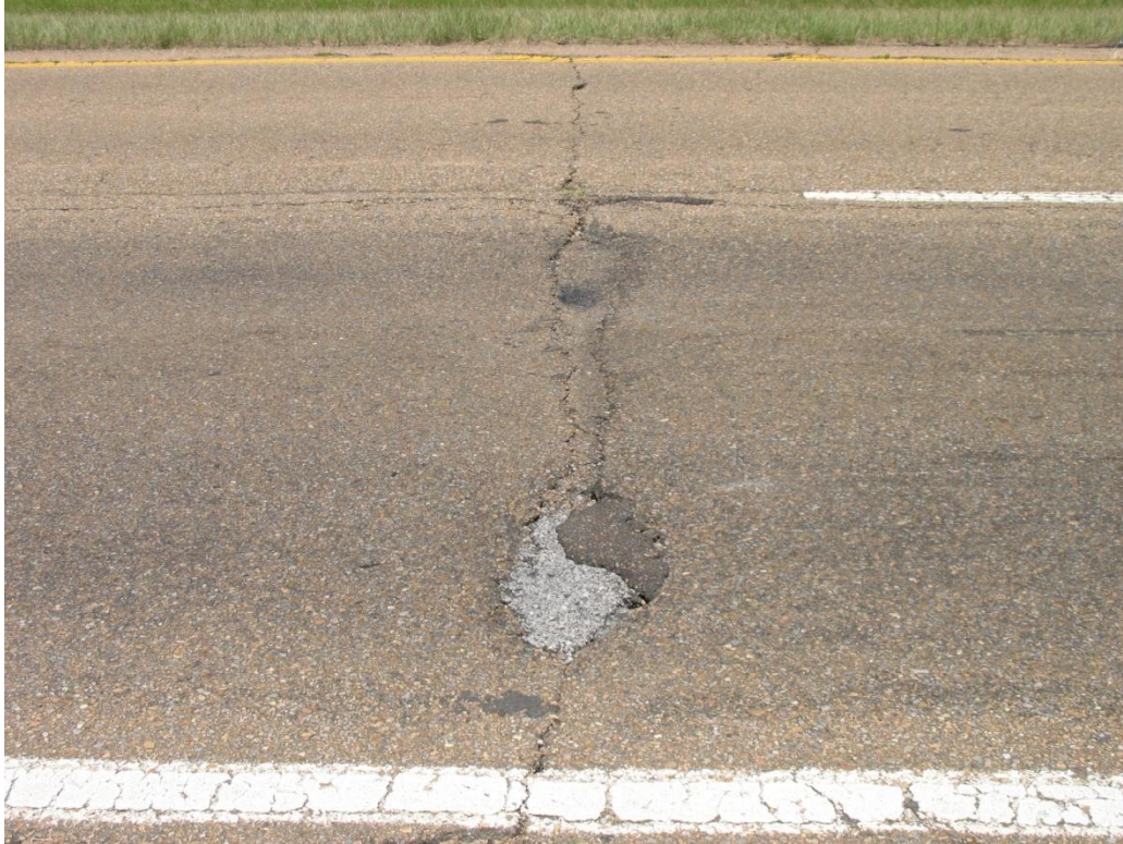
Figure 5: Transverse Cracking/Spalling
