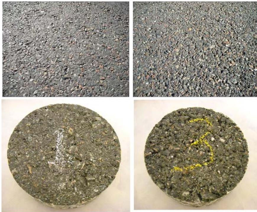
Figure 7. Russell County Pavement Sections and Specimens
