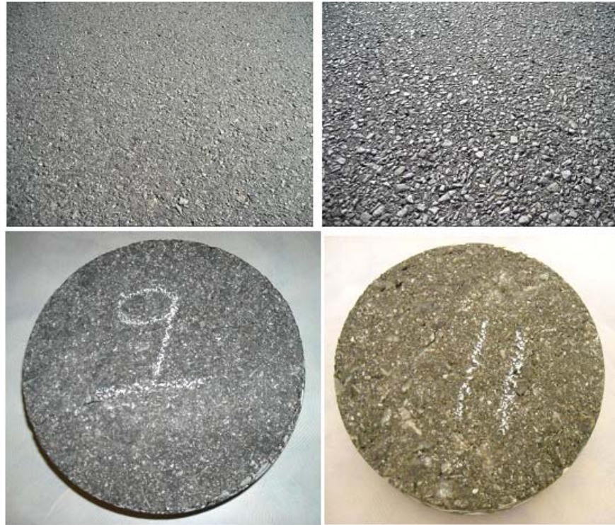
Figure 8. Tazewell County Pavement Sections and Specimens
