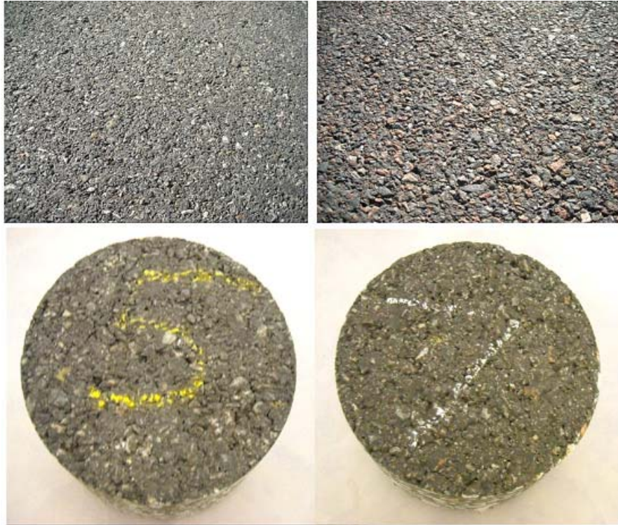
Figure 6. Buchanan County Pavement Sections and Specimens
