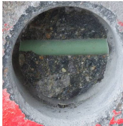
Figure 66. Structure 2900, Bent 32, Pile A, Epoxy-Coated Reinforcing Wrap
