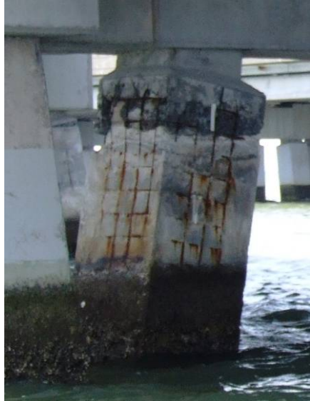
Figure 62. Structure 2902, Bent 23, Pile C
