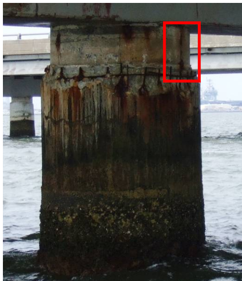
Figure 59. Structure 2900, Bent 45, Pile B, Prior to Mortar Demolition
