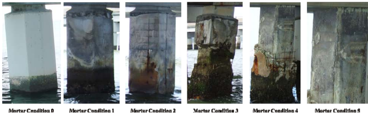
Figure 11. Visual Condition Rating of Mortar. The ratings are described in Table 2.
