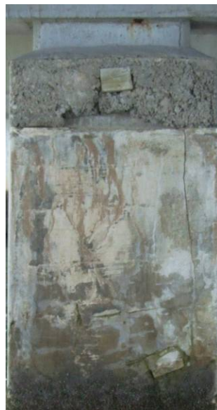
Figure 19. Mortar with Wood Blocks
