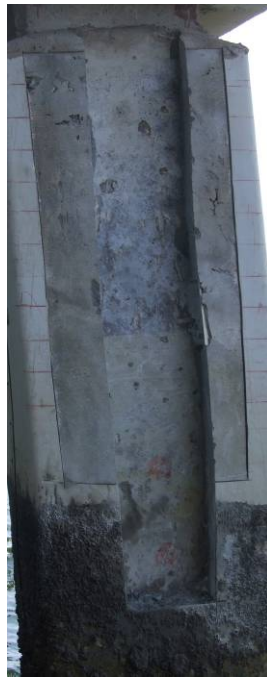
Figure 55. Structure 2866, Bent 67, Pile H
