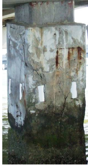
Figure 18. Mortar with Polyvinylchloride Pipe
