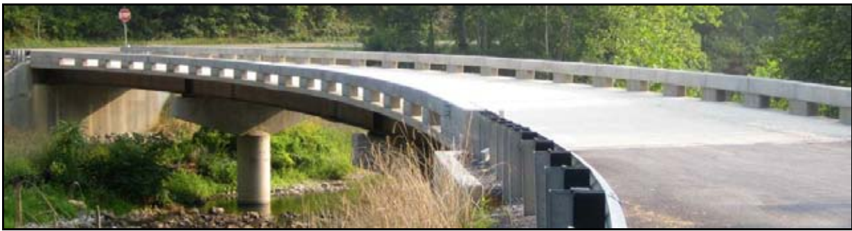
Figure 1. Wolf Creek Bridge, view from the South
