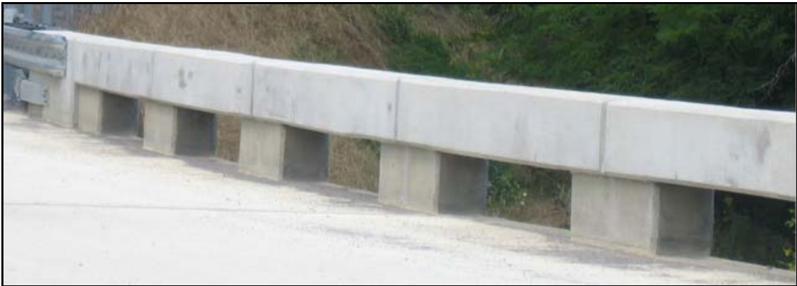
Figure 48. Railing Sections in the Field
