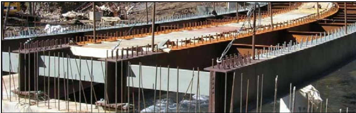
Figure 49. Shear Studs in the Field
