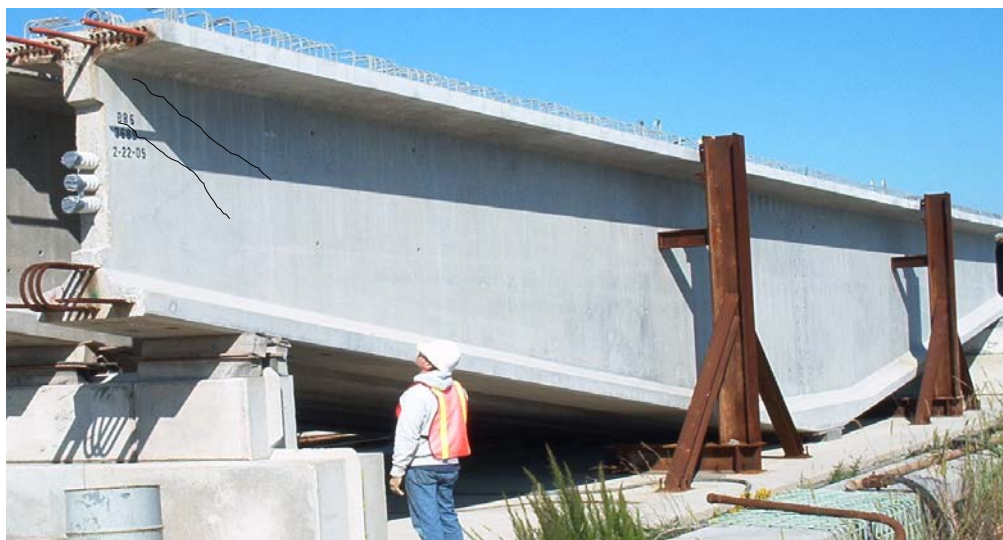
Figure 22. Anchorage Zone Cracking Observed in Deep Haunched Girders
