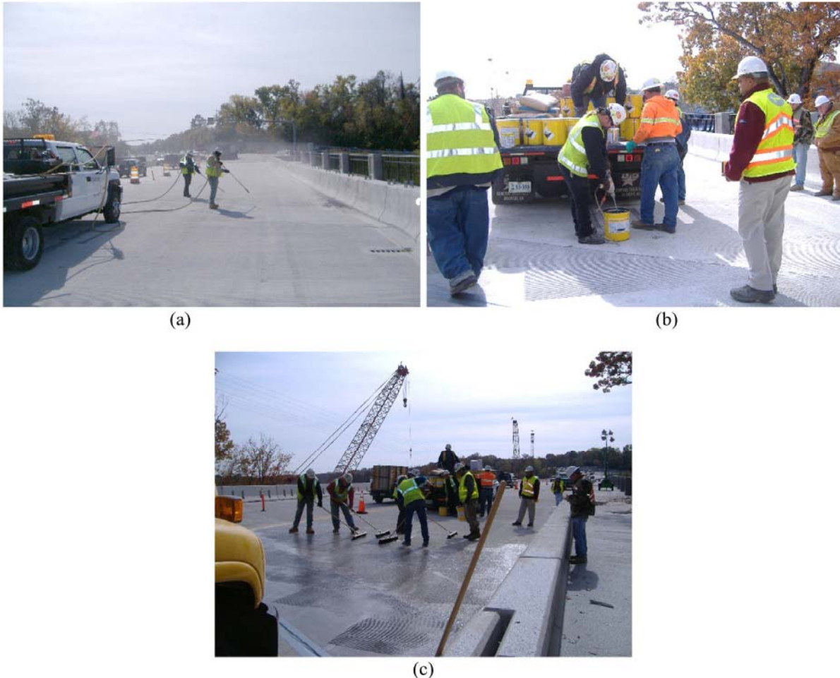
Figure 15. Crack Sealing of Southbound (ECR) Deck. (a) Cleaning of deck, (b) Mixing of epoxy, (c) Application of epoxy to deck surface.
