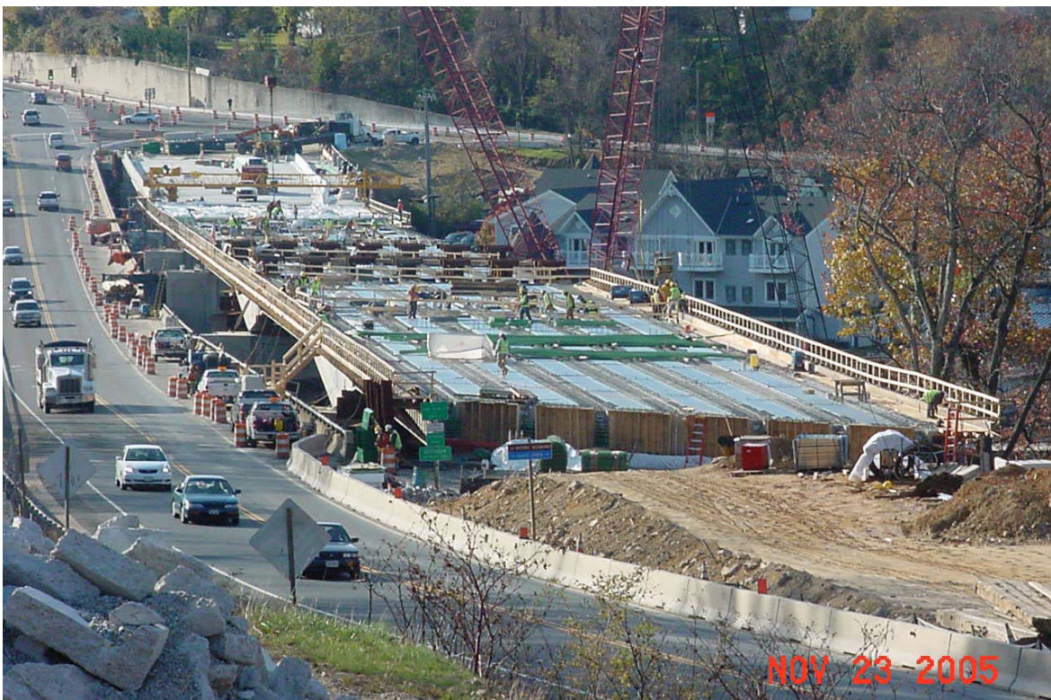
Figure 2. ECR Placement in Southbound Lane
