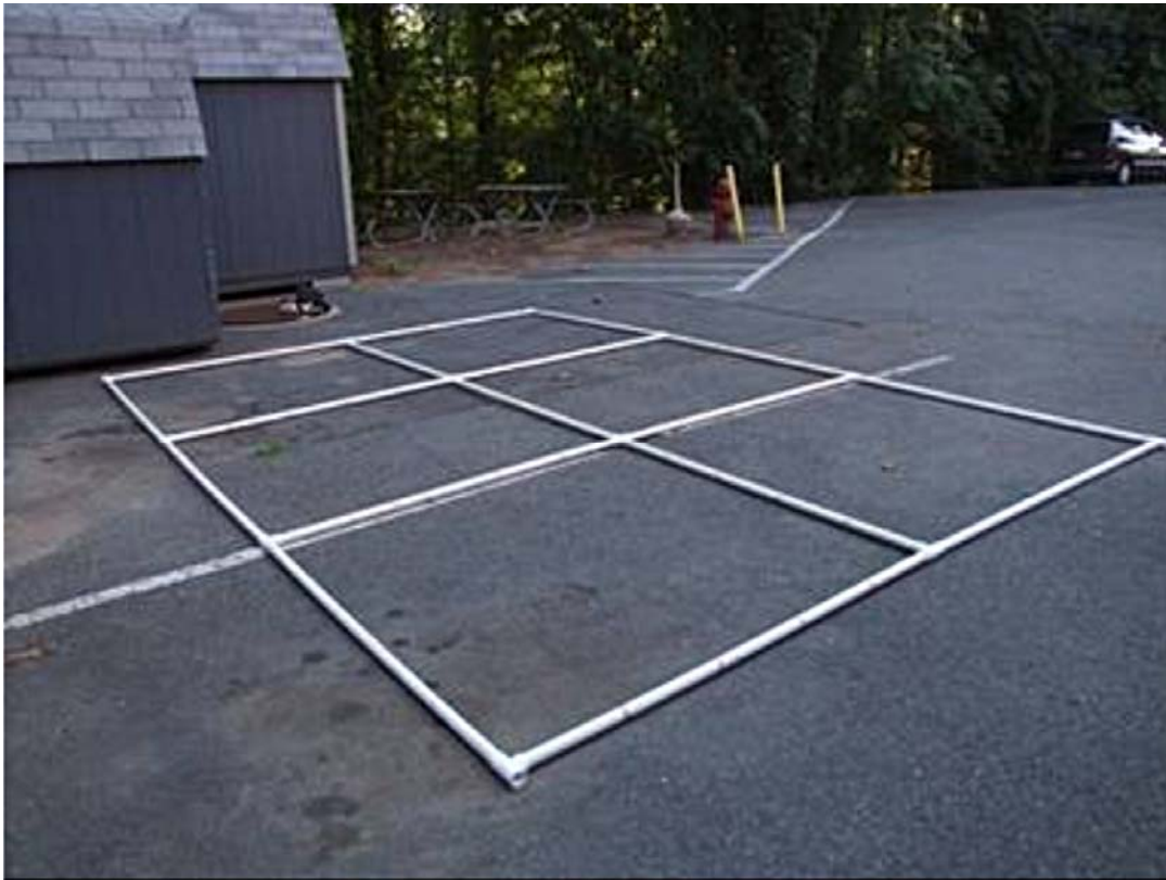
Figure 3. Crack Survey Grid
