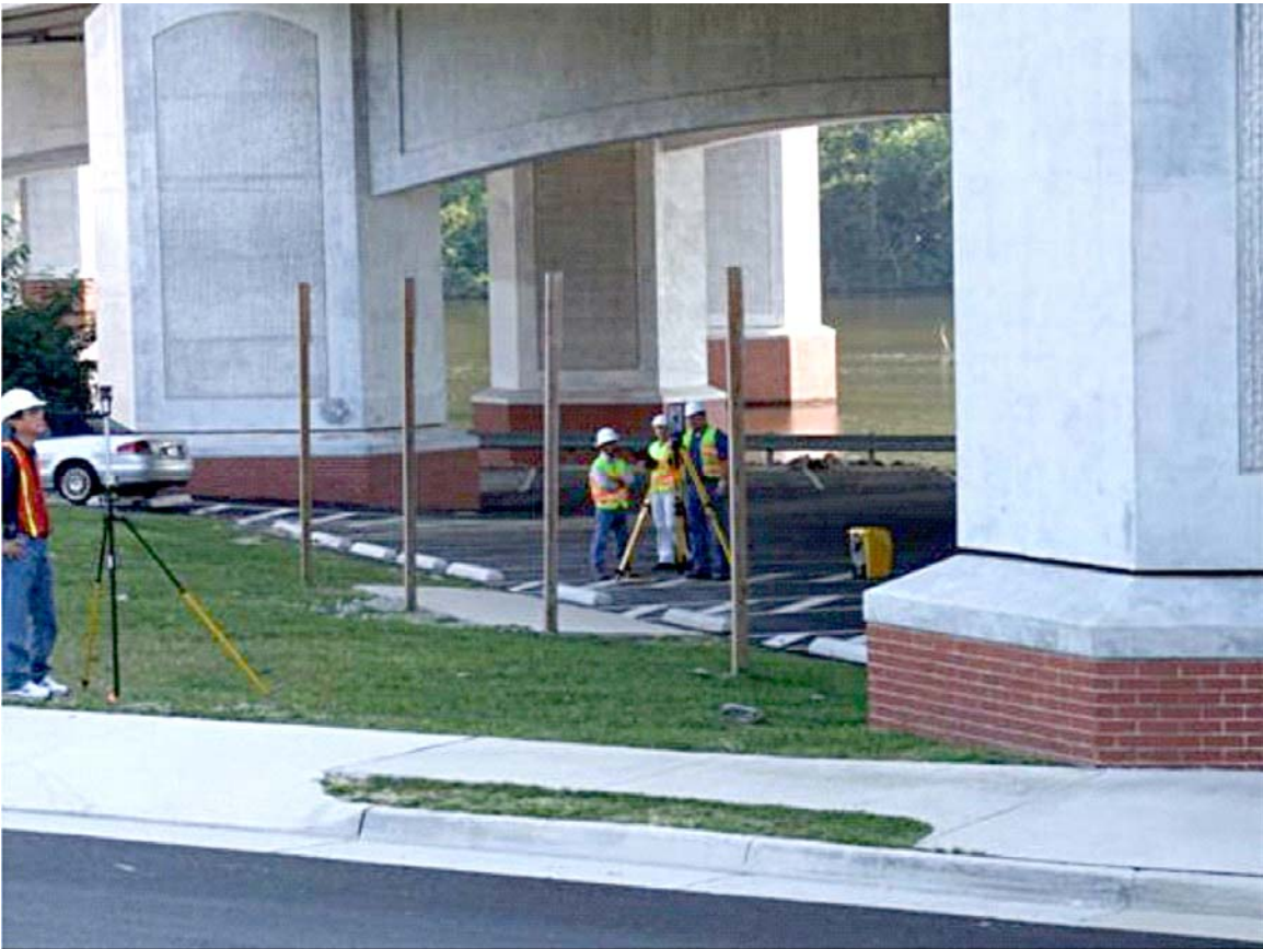
Figure 4. Gathering Coordinates to Locate Trimble VX System for Under-Bridge Crack Survey
