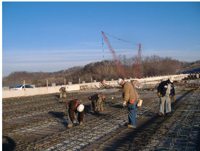
Figure 34. Walkways Not Required Over MMFX 2
