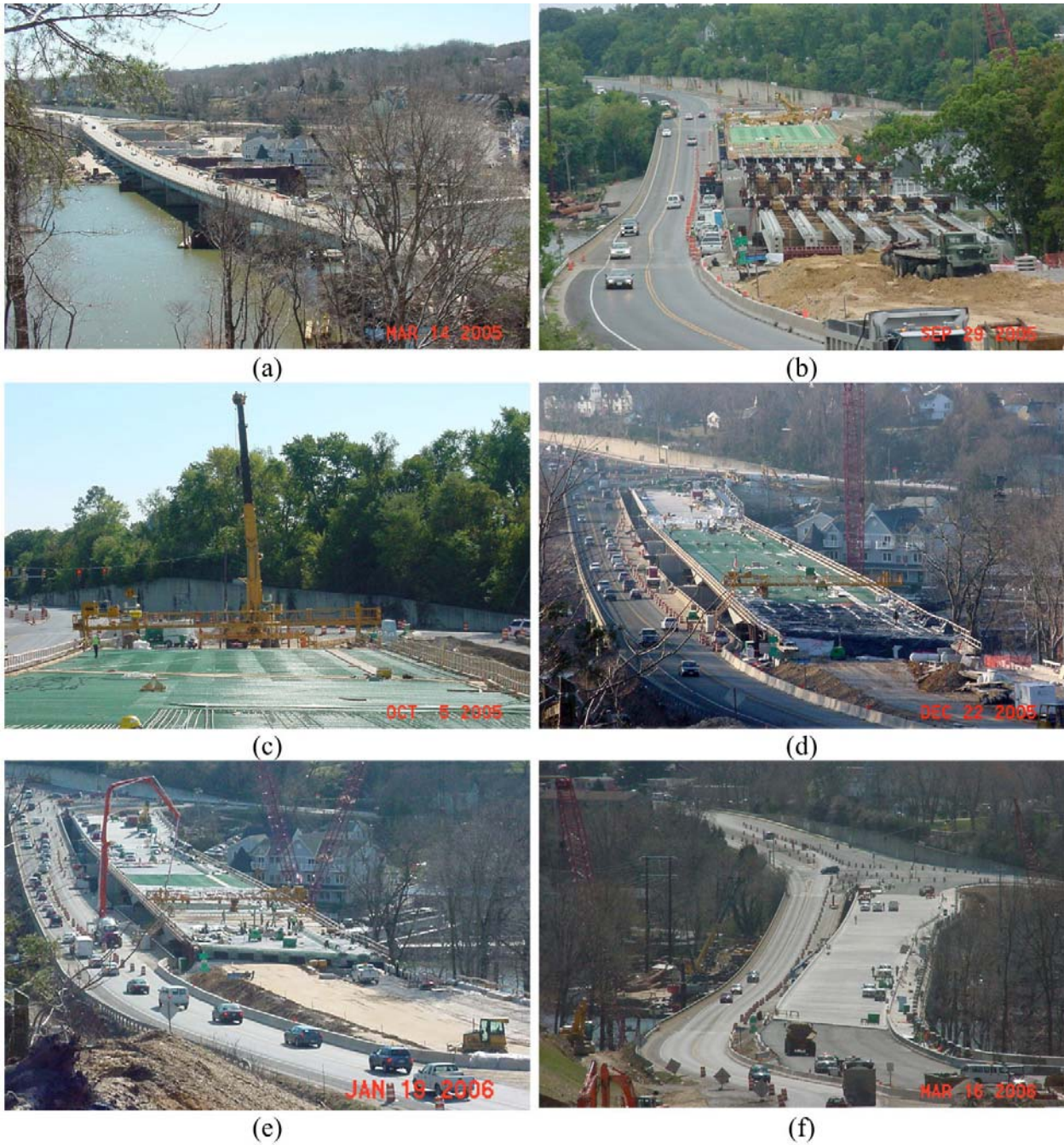
Figure 10. Construction of Southbound (ECR) Deck. (a) Substructure under construction, (b) ECR on southern end of deck, (c) Close-up of deck, (d) ECR placement near completion, (e) Placement of concrete in deck, (f) Concrete placement complete.
