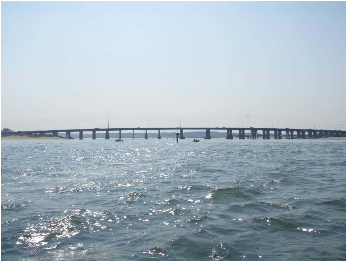
Figure 2. North Elevation of Lynnhaven Bridge 5
