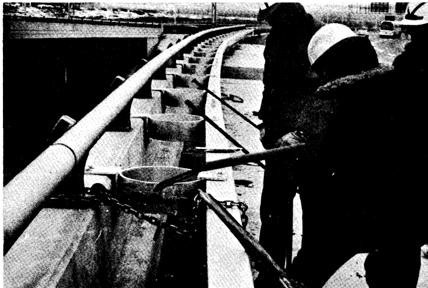
Figure 12. Attaching rail to collapsible ring support. Force was required due to presence of weld, Figure 11.
