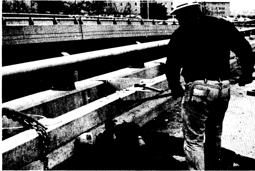
Figure 15. Completing rail splice.
