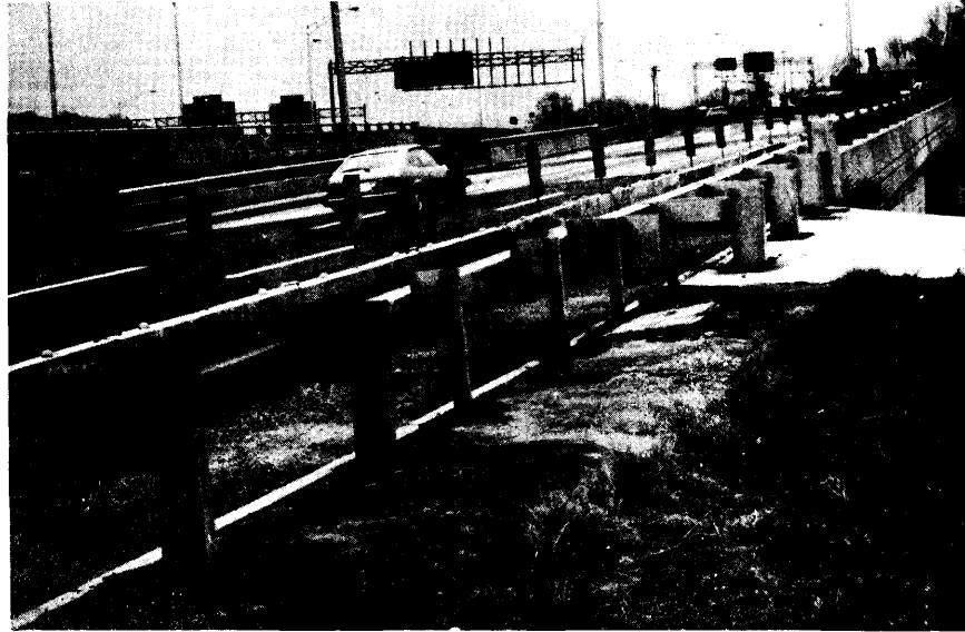
Figure 1. View of the transition between the W-beam approach guardrail (left) and bridge rail at the entry to the structure.
