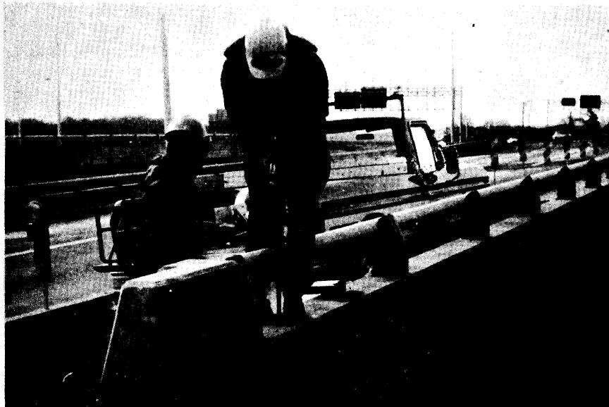
Figure 6. Drilling holes for support bolts, top face of parapet.
