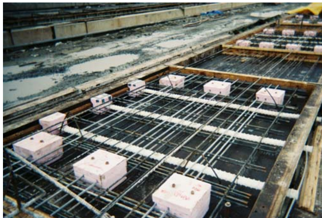
Figure 20. Layout of Stressing Bed for Precast Panels.
