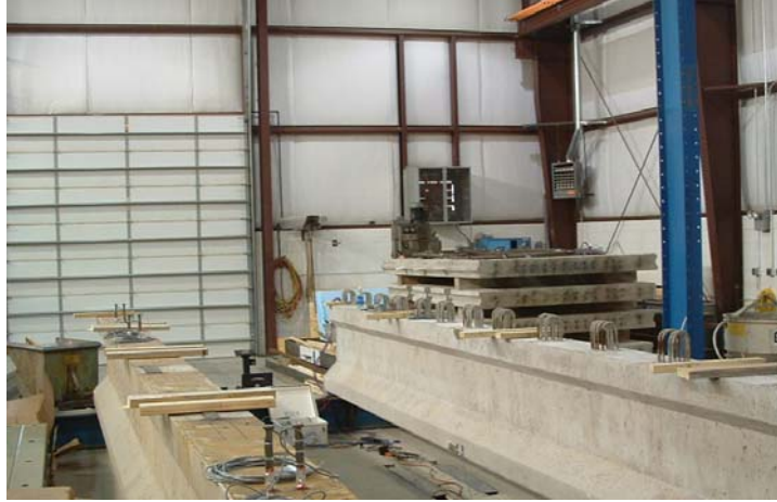
Figure 22. Girders with Wood Blocks in Place for Panel Erection.
