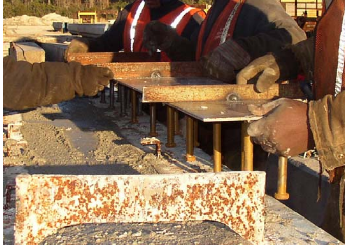
Figure 2. New Detail For Horizontal Shear Reinforcement.
