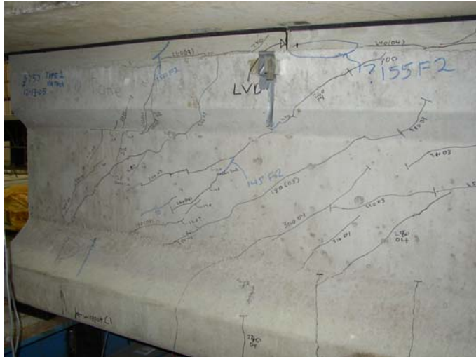
Figure 43. Cracking Pattern at Dead End for Girder 1 During Final Static Test.
