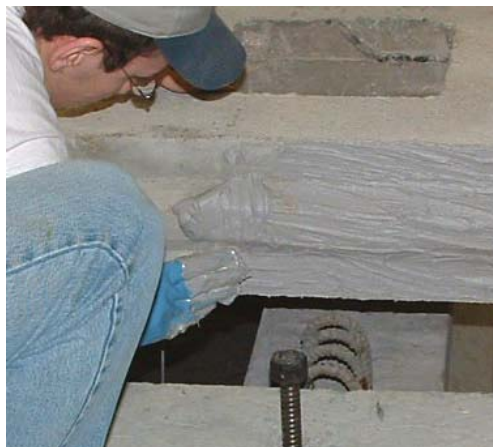
Figure 25. Epoxy Being Placed on Male-Female Joint.
