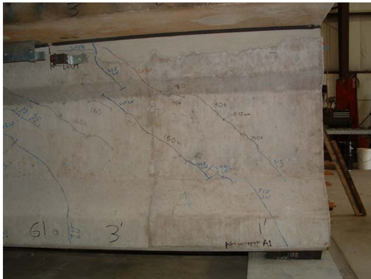
Figure 49. Cracking Pattern at Live End for Girder 1 During Final Static Test.
