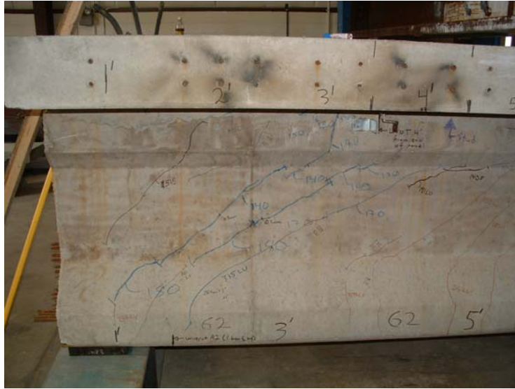
Figure 50. Cracking Pattern at Live End for Girder 2 During Final Static Test.
