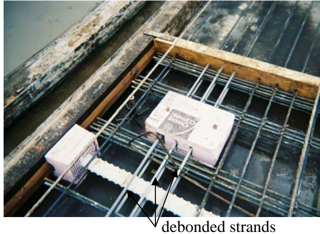
Figure 21. Formwork for Transverse Joint.
