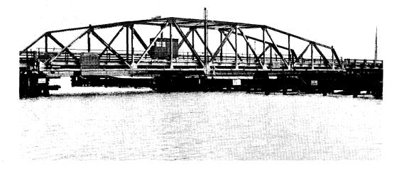
Figure 11. The Pungo Ferry Bridge in Virginia Beach is a bobtailed swing span.
