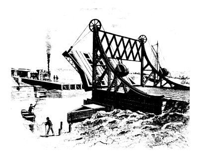
Figure 3. An example of an early counterweighted bascule bridge.
