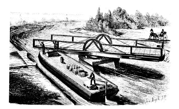
Figure 9. A wooden swing bridge patented by John Selser in 1861.
