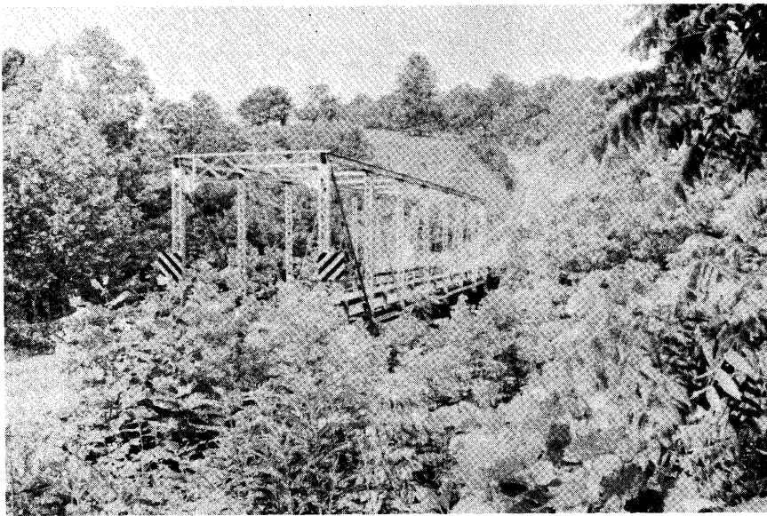
Figure 7. The only true bedstead/leg truss surveyed in Virginia, located in Bedford County. (Bedford Co., photo #12455-14-2A)
