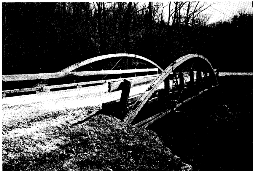
Figure 6. Virginia's oldest extant metal truss bridge, the relocated Bedford County bowstring truss. This King Co. truss is now located in Montgomery County and is used as a pedestrian bridge. (Montgomery Co., photo #11916)
