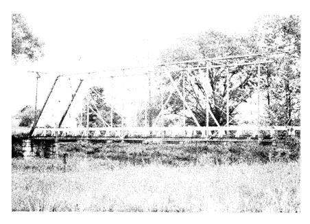
Figure 14. Whipple-type truss, Rockingham County; built by the Wrought Iron Bridge Company, Canton, Ohio, in 1898. (See form/photo number 08-81-35.)
