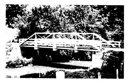
Figure 6. A typical pin connected Low/Pony truss used for a 58-foot span bridge. (Rockingham County; see form/photo number 08-82-7.)
