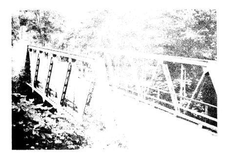
Figure 11. A Low Triangular/Warren-type truss span featuring rigid connection details. (Augusta County; see form/photo number 08-07-4.)
