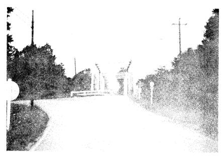
Figure 18. Two-span Pratt truss bridge in Rockbridge County having 30<sup>o</sup> skew; built by the Groton Bridge & Manufacturing Company, Groton, New York, in 1890. (See form/photo number 08-81-6.)
