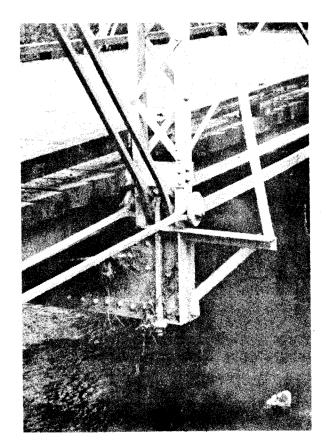
Figure 9. A pin connection at a truss panel point, the junction of an intermediate post, a top or bottom chord member and several diagonals. (Rockbridge County; see form/photo number 08-81-15.)
