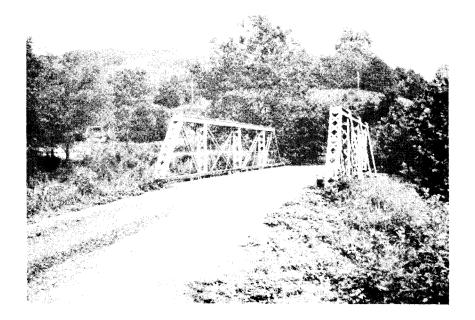
Figure 21. Single-span, low Pratt, half-hip truss bridge in Rockbridge County; built by Variety Iron Works, Cleveland, Ohio; date unknown. (See form/photo number 08-81-15.)
