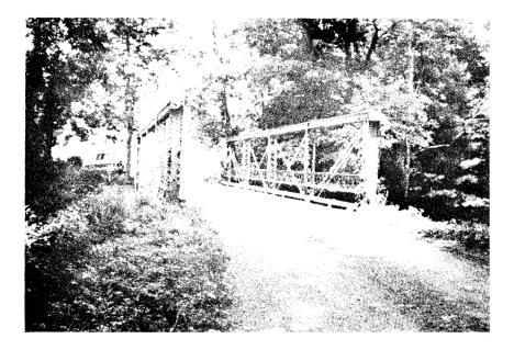
Figure 20. One of five bedstead/truss leg bridges built in the Staunton Construction District; dates unknown. (See form/photo number 08-07-13.)
