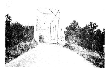
Figure 17. Three-span quadrangular truss bridge in Rockingham County and possibly constructed in 1903; builder unknown. (See form/photo number 08-82-36.)
