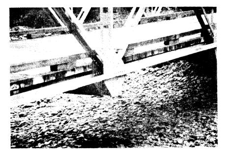
Figure 10. A rigid connection featuring a gusset plate to which are riveted the intersecting chord members, post angles, and the several diagonals. (Rockingham County; see form/photo number 08-82-3.) هنكا براكان وقدر
