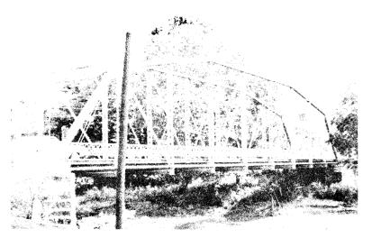
Figure 8. A typical Through Camelback truss bridge whose inclined top chords rendered it more economical for exceptionally long spans; span length 150 feet. (Augusta County; see form/ photo number 08-07-27.)
