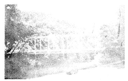
Figure 7. A typical Through/High truss bridge having a span length of 115 feet. (Augusta County; see form/photo number 08-07-21.)
