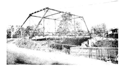
Figure 19. Single-span Pratt truss bridge in Covington, Virginia; built by the Phoenix Bridge Company; the date is unknown. (See form/photo number 08-81-7.)
