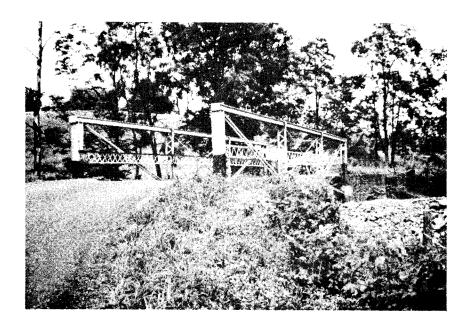
Figure 13. A typical low Bedstead/Truss Leg truss configuration with vertical end posts. (Augusta County; see form/photo number 08-07-15.)
