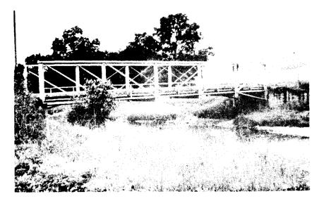
Figure 3. A low Truss Leg bridge with the less satisfactory vertical end posts. (Augusta County; see form/photo number 08-07-14.)
