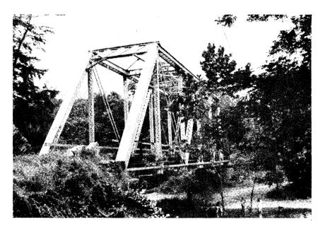
Figure 16. Single span triangular/Warren-type truss in Augusta County with pin connections. Builder and date unknown. (See form/photo number 08-07-30.)
