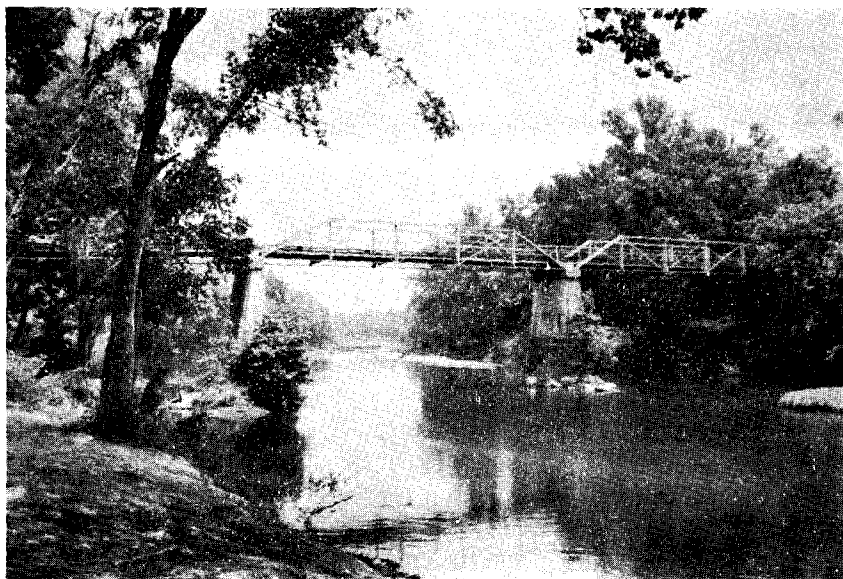
Figure 11. Five-span, low/pony Pratt truss, full-slope bridge built by the Horseheads Bridge Company, Horseheads, New York, in 1898. (Culpeper-Fauquier County line, see form/photo number 07-23-2.)
