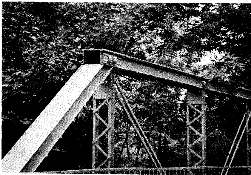
Figure 15. Single-span, low/pony Pratt truss, full-slope with unusual butt end at top chord/end post panel point; builder and date unknown. (Loudoun County, see form/photo number 07-53-1.)
