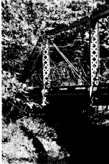
Figure 8. Latticing used on posts. (Rappahannock County, form/photo number 07-78-3.)
