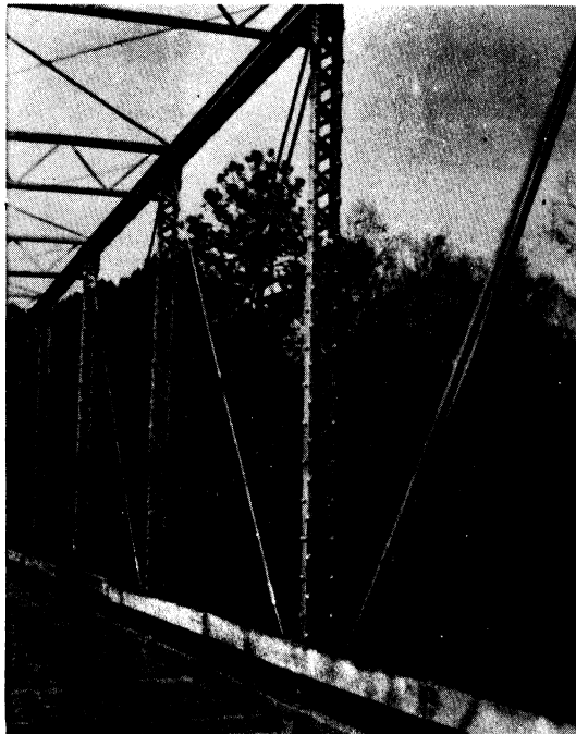
Figure 9. Lacing bars used on posts and lateral struts of a through/high Pratt-type truss built by Virginia Bridge and Iron Company, Roanoke, Virginia; date unknown. (Dinwiddie/Brunswick County line; form/photo number 04-26-1.)
