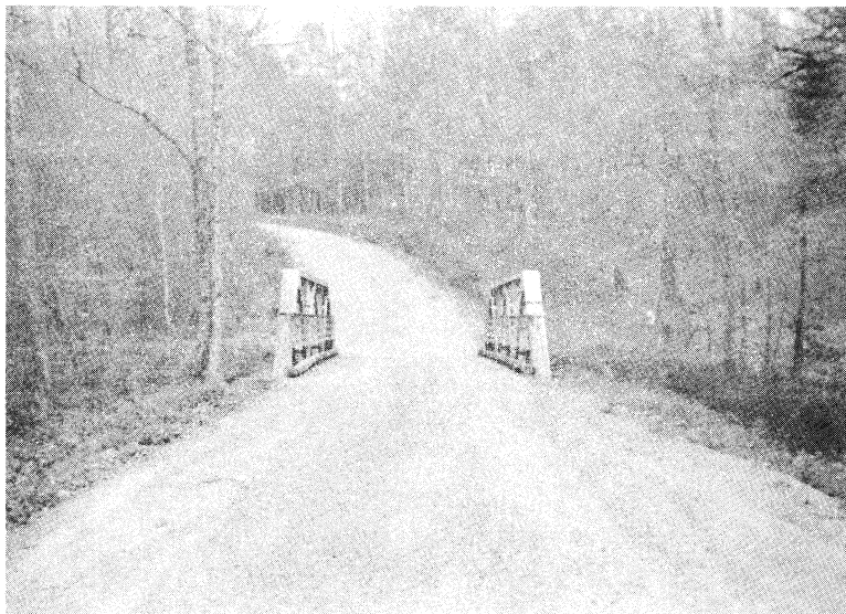
Figure 7. Single-span low/pony triangular truss with a 46-foot span built in 1913 by the York Bridge Company, York, Pennsylvania. (Mecklenburg County; form/photo number 04-58-4.)
