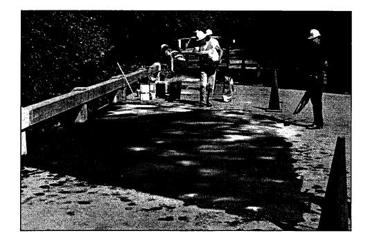
Figure 106. Sand must be broadcast onto the resin to provide an acceptable skid number. The sand may be omitted if the resin is applied to a grooved or tined surface, but care must be taken to ensure that the resin does not fill the grooves.
