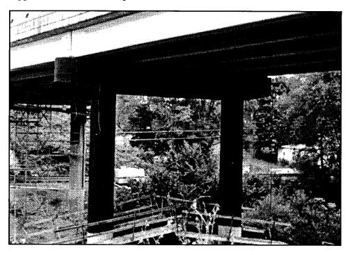
Figure 189. A conductive coating has been applied to the piers and bent to provide applied current cathodic protection.
