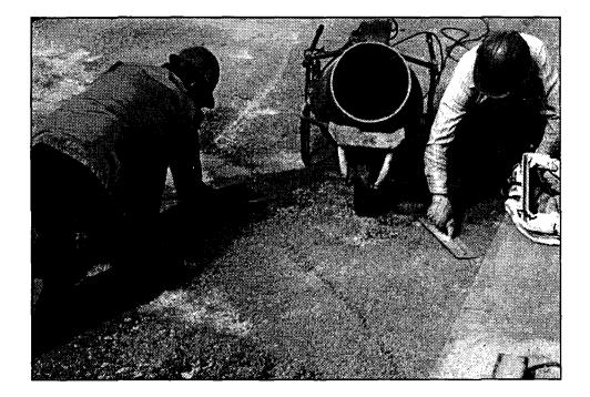
Figure 73. Areas to be patched with epoxy mortar shall be dry and shall be primed with neat epoxy prior to placing the mortar.
