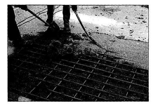
Figure 84. Very rapid hardening hydraulic cement concrete may appear stiff prior to being consolidated. Internal vibration rather than additional mix water should be used to achieve good consolidation of the concrete.
