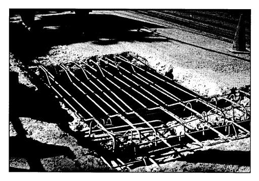
Figure 75. Type C patches (full depth) require forms to be suspended from reinforcing steel (areas <3 ft<sup>2</sup>) or supported by blocking from beam flanges.
