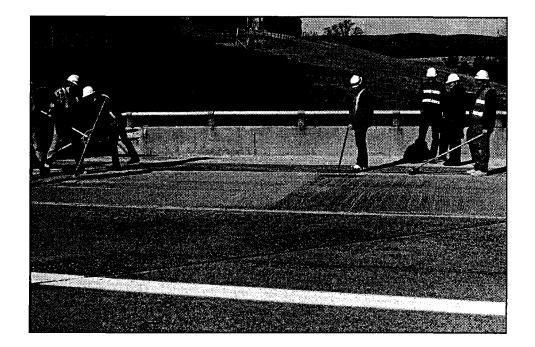
Figure 132. The latex-modified hydraulic cement slurry is tined with 1/8 in. wide by 1/8 in. deep grooves spaced 3/4 in. on center to provide a skid resistant surface.
