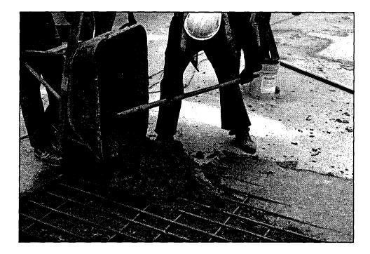
Figure 82. The mixed concrete is usually transported to the patch site with a wheelbarrow. Internal spud vibrators must be used to consolidate the concrete. The mixture should have a slump of 2 to 4 in. and should not segregate when consolidated. The hardened concrete surface should be wetted to achieve a saturated-surface-dry condition prior to placing the fresh concrete.
