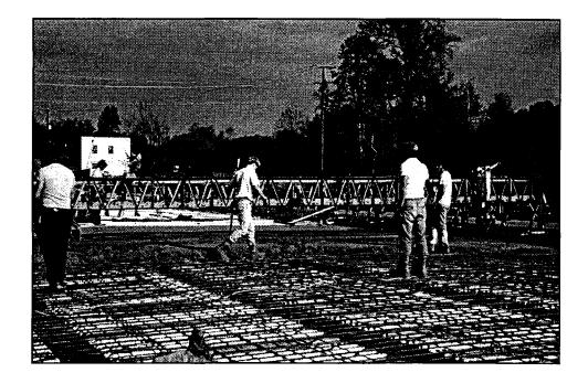
Figure 98. Placement of concrete to widen a bridge deck. Silica fume, fly ash and slag are being used in concrete to reduce the lifecycle costs, to obtain high early strengths (silica fume), and to utilize materials that might have to be placed in landfills.
