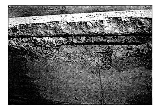
Figure 48. Prestressed strands are corroded and concrete is not properly consolidated in spalled areas of beam.
