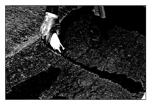
Figure 107. High molecular weight methacrylate can be applied to a crack. For satisfactory filling of the crack, it should be free of debris and wider than 0.1 mm. Also, best results can be obtained by filling cracks when they are open the widest at the surface (temperatures between 55°F and 70°F and between 1:00 a.m. and 10:00 a.m). High molecular weight methacrylate will not cure satisfactorily at temperatures below 55°F.
