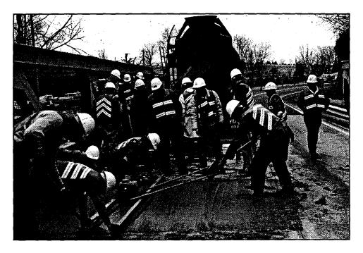
Figure 79. The hydraulic cement concrete shall be properly consolidated with internal vibrators and a vibrating screed may be used to strike off the surface.
