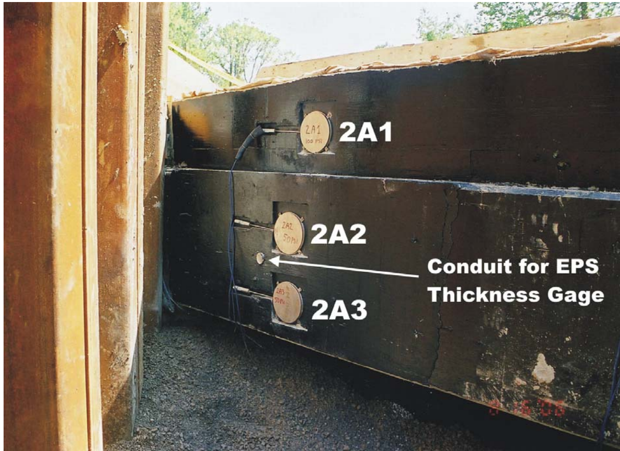
Figure 11. Elevation View of Some Pressure Cells at Abutment A
