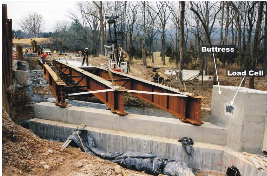
Figure 6. Concrete Butress at Abutment B
