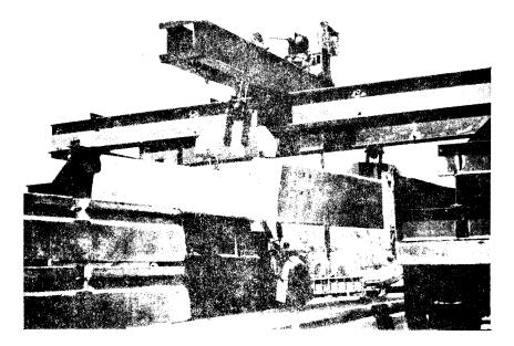
Figure 16. Gantry crane moving preclass that from storage area to trailer.
