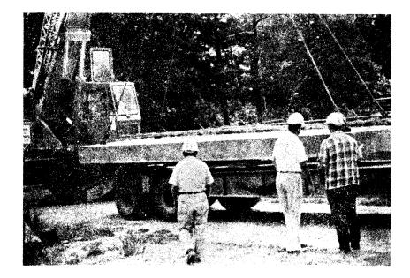
Figure 15. Truck crane lifting precast slab.
