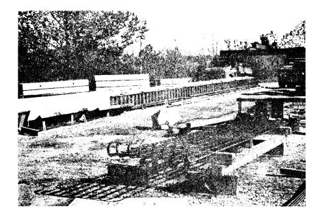
Figure 17. Slabs in storage at Staunton District casting yard.
