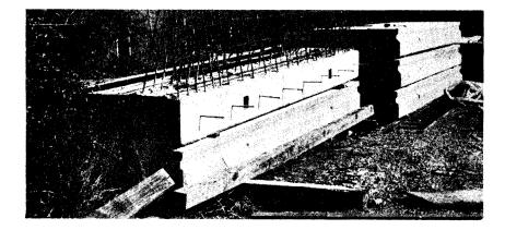
Figure 9. Exterior beam with all the parapet steel cast in slab.
