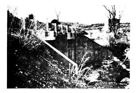
Figure 4. Two-span precast slab bridge on Rte. 724 near Harrisonburg.
