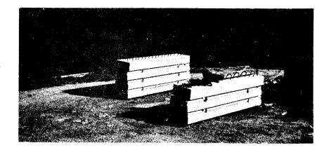
Figure 10. Exterior beam with a few large parapet bars cast in slab.
