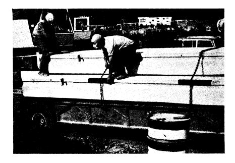
Figure 18. Three slabs properly secured to lowboy trailer.
