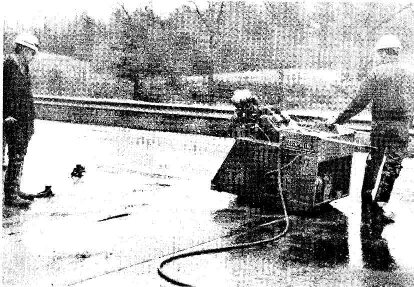
Figure 19. Full-depth sawing of repair limits.
