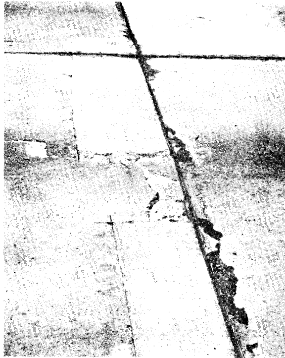
Figure 6. Continued deterioration of concrete in foreground occurred after full-depth restoration of lane in background.
