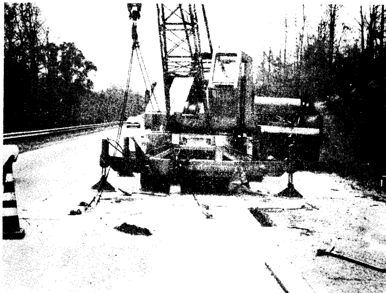
Figure 27. Precast slab in place.
