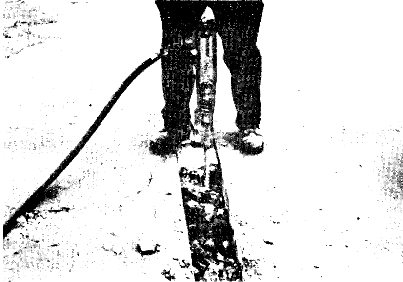
Figure 21. Stress relief at one end of repair area requiring third transverse sawcut (Michigan photo).
