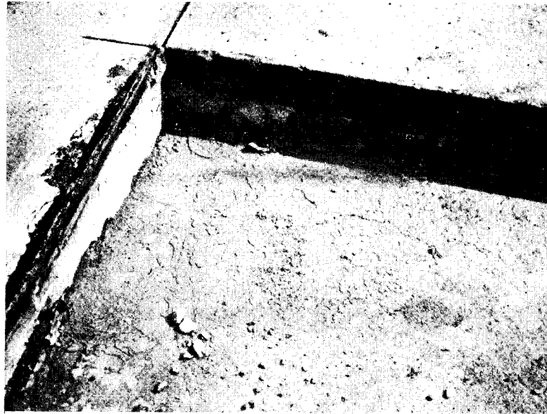
Figure 31. Fine subbase material infiltrated between mortar layer and precast slab from underneath adjacent roadway areas (roadway centerline on left).
