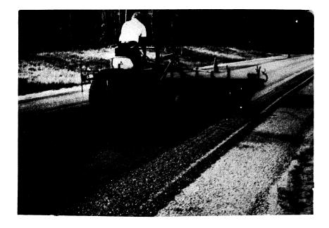
Figure 2. Tractor placing Petromat and resulting wrinkles in fabric.
