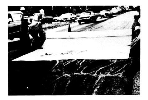
Figure 3. Mirafi being placed with the aid of hand brakes.
