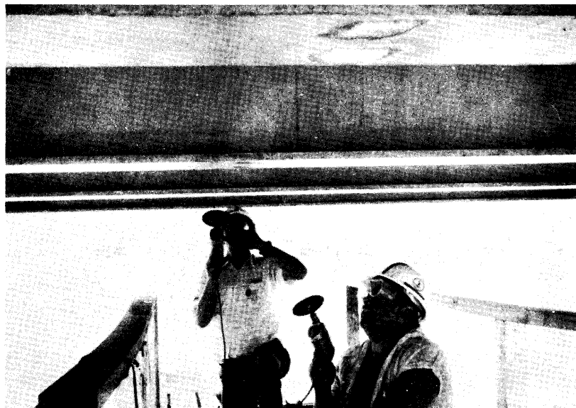
Figure 11. Grinding of surfaces of steel girders in preparation for placing strain gages.
