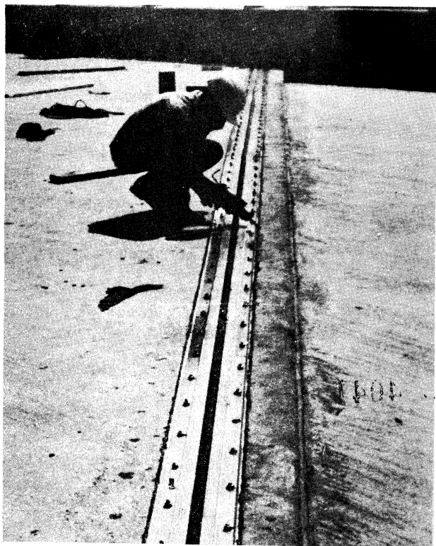
Figure 8. Applying additional sealant to the edges of the joint.
