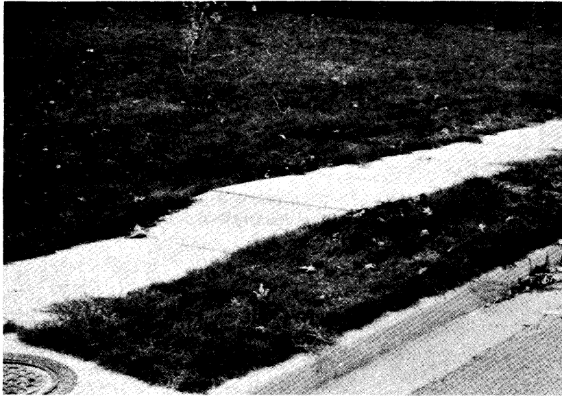
Figure 22. Uplift of sidewalk at lower end of section at Test Area #1 due to undermining upgrade of failure.
