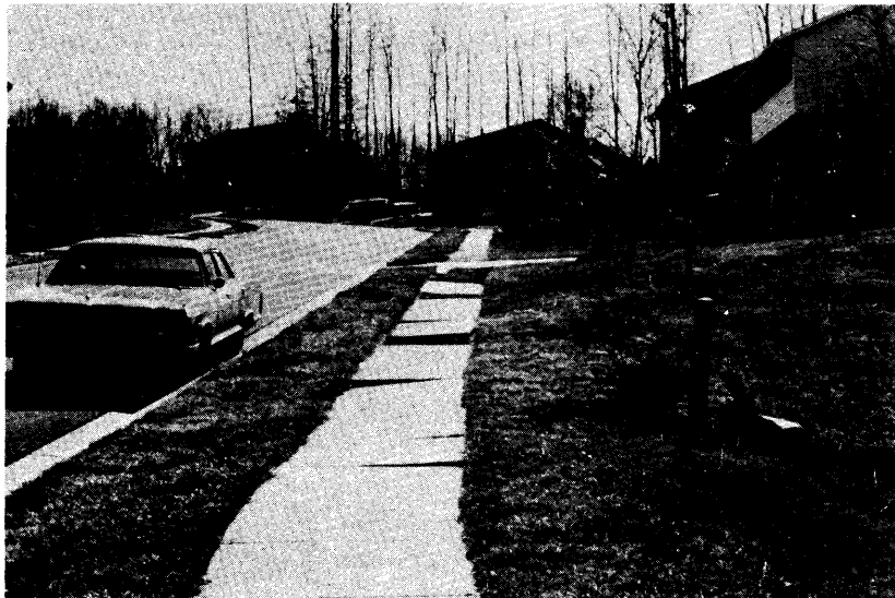
Figure 2. Severe distortion of sidewalk due to undermining.
