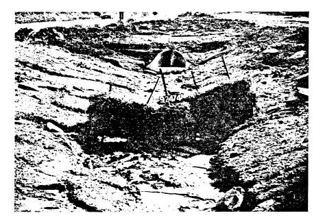
Figure 5. Severe erosion and sediment loss caused by undercutting of a straw bale barrier. Proper installation of this type of barrier will minimize failures of this type. 6. Problem: Cellulose wood fiber is generally considered to have limited effectiveness as a mulch on seeded areas.
