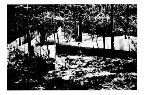
Figure 2. In areas where the cleaning of controls is costly or impractical, new barriers can be placed parallel to the old as seen here.
