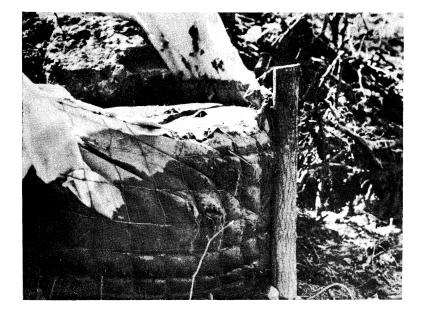
Figure 1. Silt fence filter barrier filled with sediment. Trap efficiency is greatly reduced.
