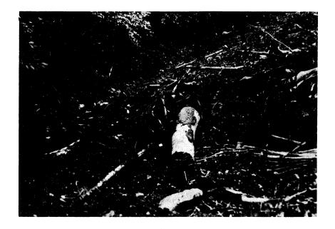
Figure 6. Brush and root mat barrier windrowed at the toe of a fill.
