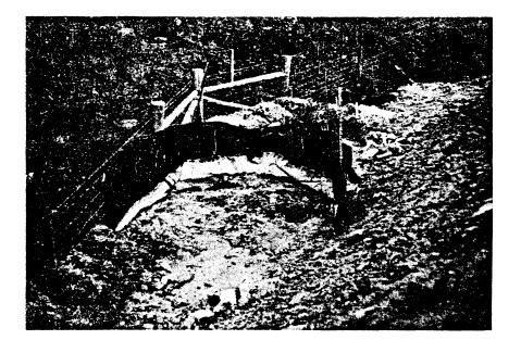
Figure 3. Filter fabric silt fence working well. However, lack of access for equipment will likely make cleaning of fence difficult and costly.
