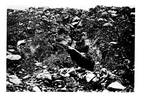
Figure 10. Erosion attributable to a lack of inspection on berms and down drains.
