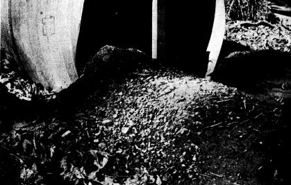
Figure 7. Accumulation of sediment in drain pipe at outlet end. Placing pipe at a slightly higher elevation would help eliminate this harmful buildup of sediment.
