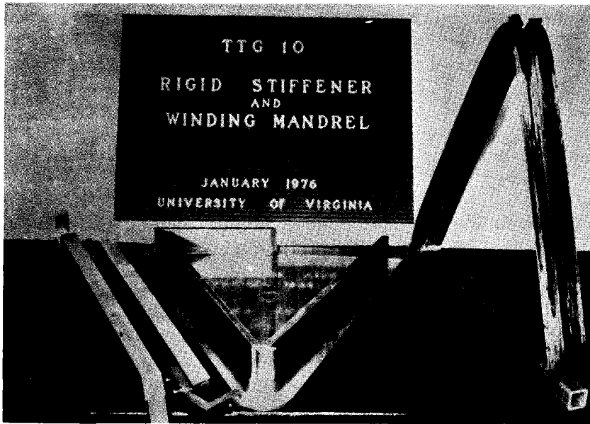
Figure 6. View of finished rigid stiffener and disassembled mandrel used for filament winding the stiffener.
