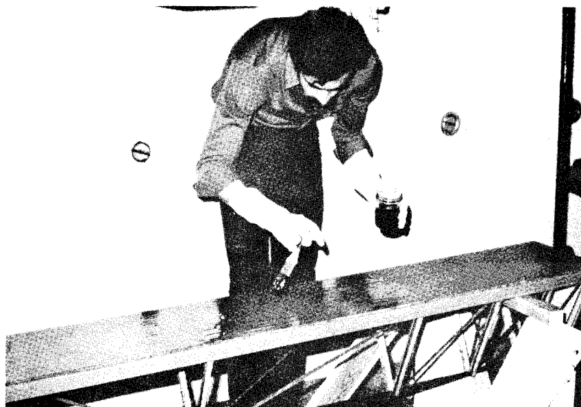
Figure 8. Application of resin binder for top cover plate on TTG-3.
