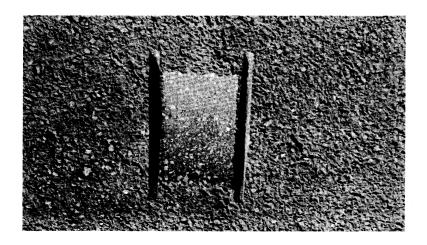
Figure 4. Pavement groove for placement of casting and markers.
