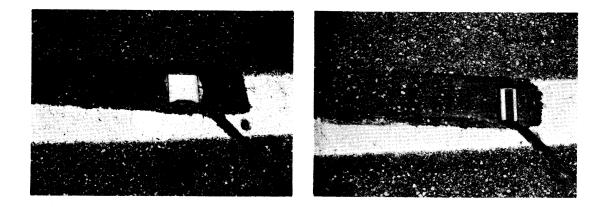
Figure 1. Markers (reflecting unit only) placed in grooves along pavement edge.
