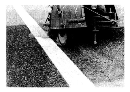
Figure 6. Groove being cut in pavement.
