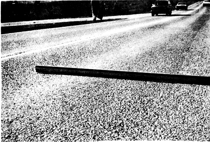
Figure 8. Limestone mix on Route 114, Montgomery County.
