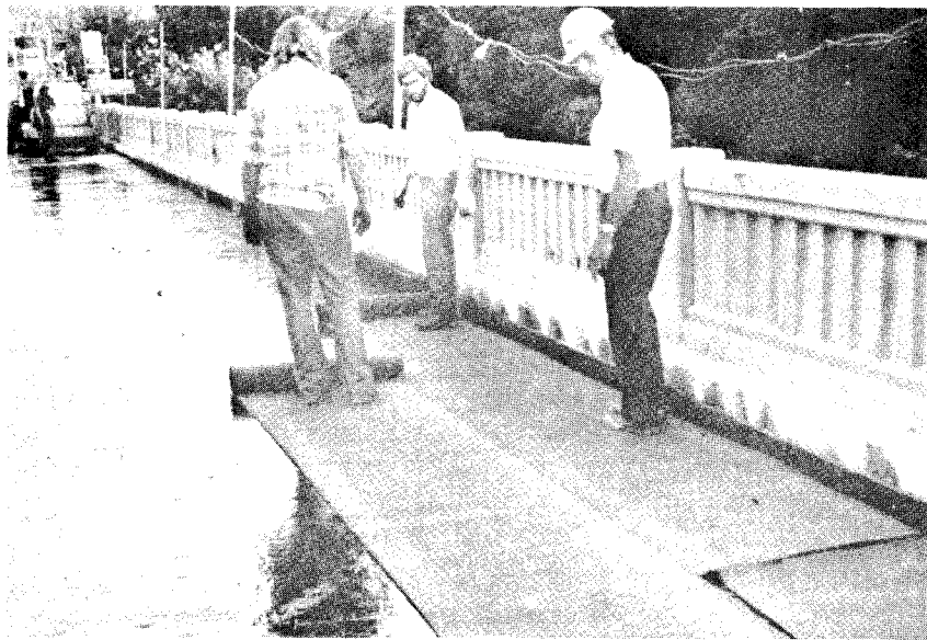
Figure 19. Placement of roofing sheet on Polytok membrane.
