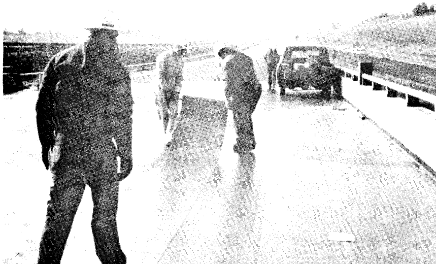
Figure 10. Unrolling of Protecto-Wrap membrane.
