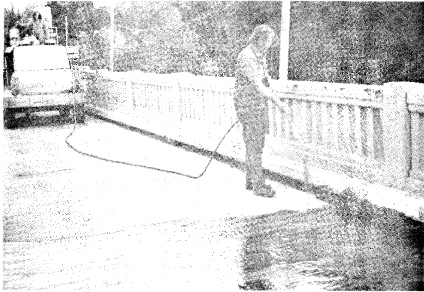
Figure 18. Spray application of Polytok liquid membrane.
