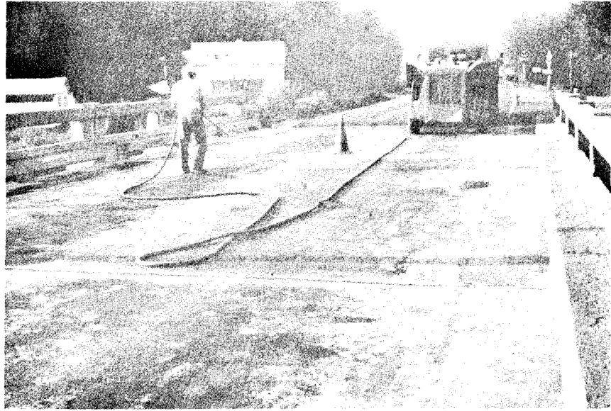
Figure 4. Deck surface prepared for application of Bituthene membrane
