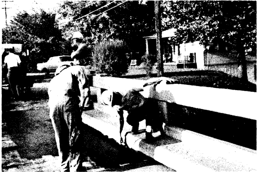
Figure 5. Application of Bituthene primer.
