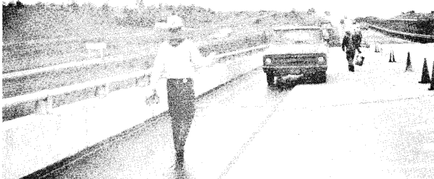
Figure 11. Rolling with light truck to set the laps between adjacent membrane sheets.
