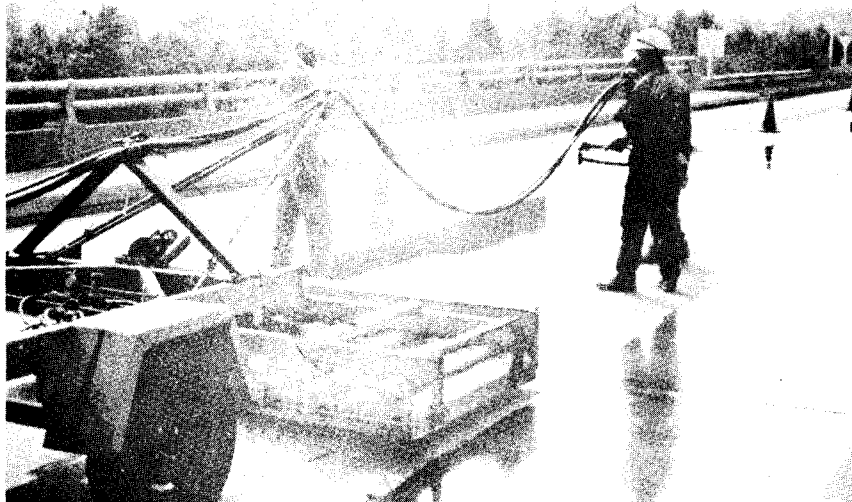
Figure 22. Spray application of Chevron's membrane system.
