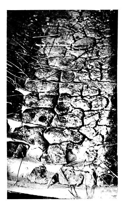
Figure 2. Widening of cracks in the paved invert at the end of the culvert due to oxidation of the bituminous material.
