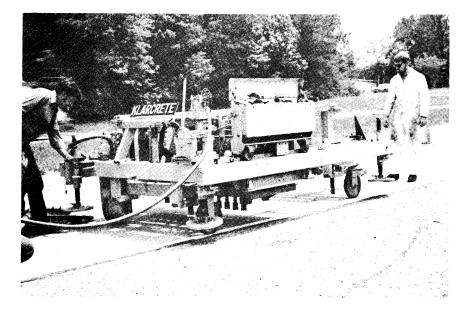
Figure 2. Klarcrete machine being positioned for operation.
