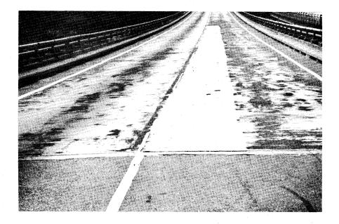
Figure 6. Cold tar epoxy on deck of northbound Meherrin River Bridge. Note single swath cleaned by Klarcrete machine.
