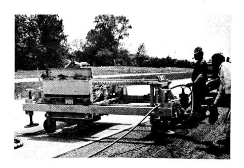
Figure 5. Klarcrete machine being turned and positioned.
