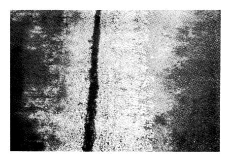
Figure 12. Concrete pavement after removal of paint lines.
