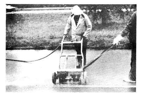
Figure 11. Paint markings being removed from concrete pavement.
