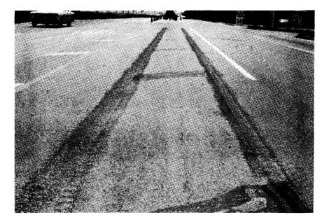
Figure 7. Accomac County pavement after removal of paint lines.
