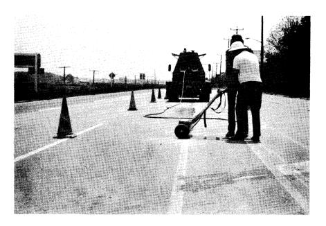
Figure 6. Removal of paint markings from bituminous pavements on Route 13 in Accomac County, Virginia.
