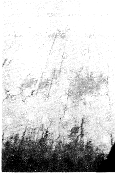
Figure 3. Typical fine transverse cracking in the DOW SM-100 latex modified mortar overlay. (NBL Interstate Rte. 85 bridge over the Roanoke River.)
