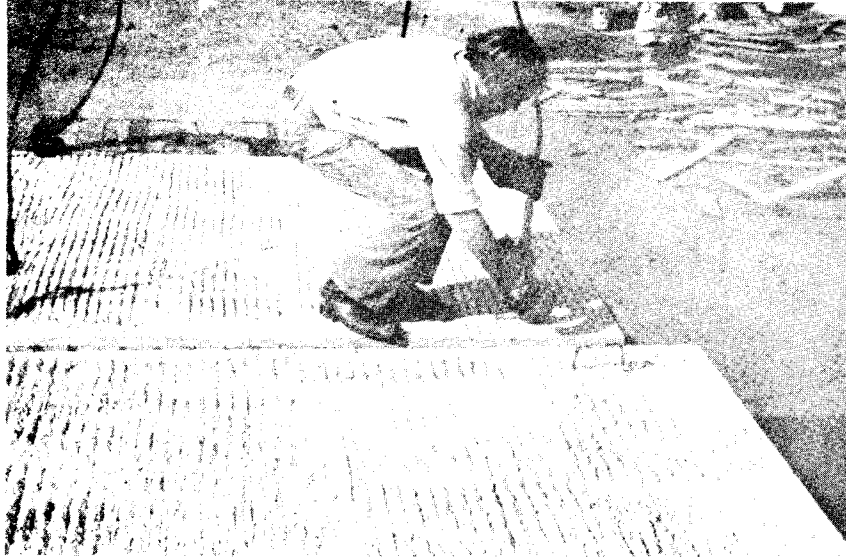
Figure 2. Prestressed panel is hooked for lifting onto the bridge superstructure.
