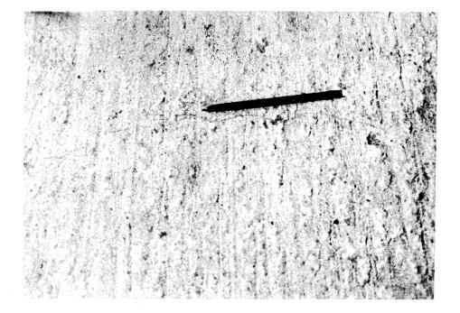
Figure 2. Typical hairline cracking observed at some locations on the surface of the bridge decks.
