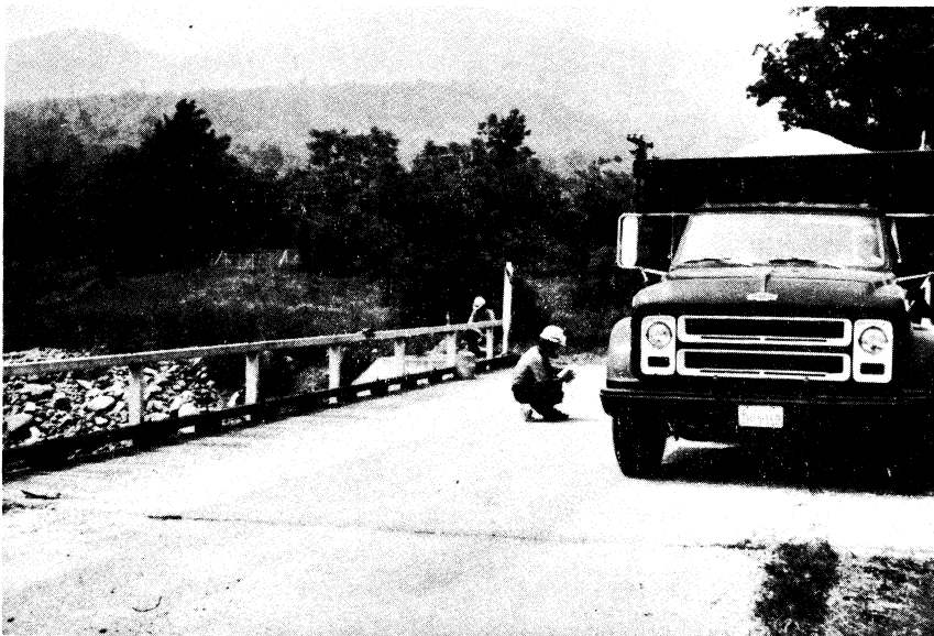
Figure 6. The truck being positioned on the 48.5 ft. timber deck span to obtain maximum moment at midspan of the steel girders.
