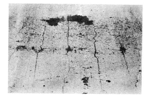
Figure 6. Recent cracking above transverse reinforcing steel in span 5. Hairline longitudinal cracking can be detected also.
